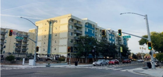
6 th /Taylor Traffic Light Installation
