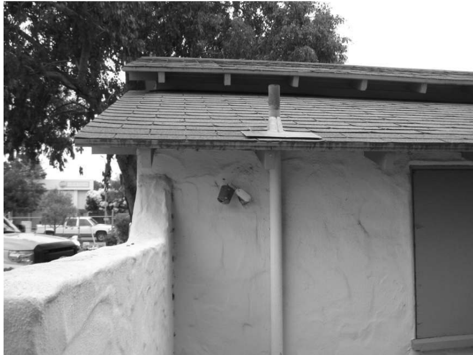
Photo 5: Detail of the western façade showing open eaves and low wall.
