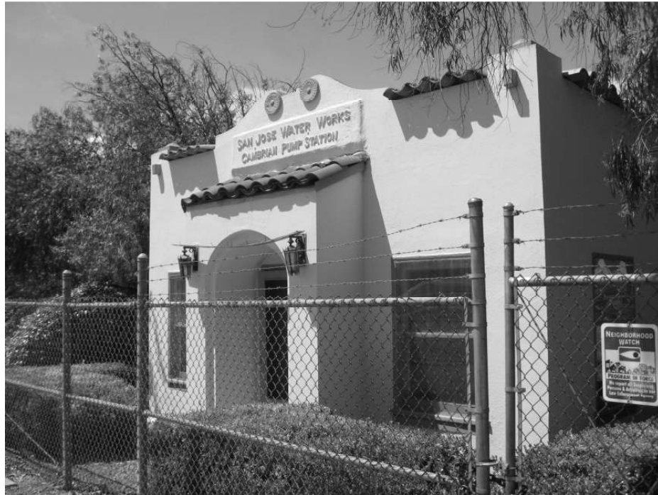
Photo 19: Oblique view of the Booster Pump Building from the north.
