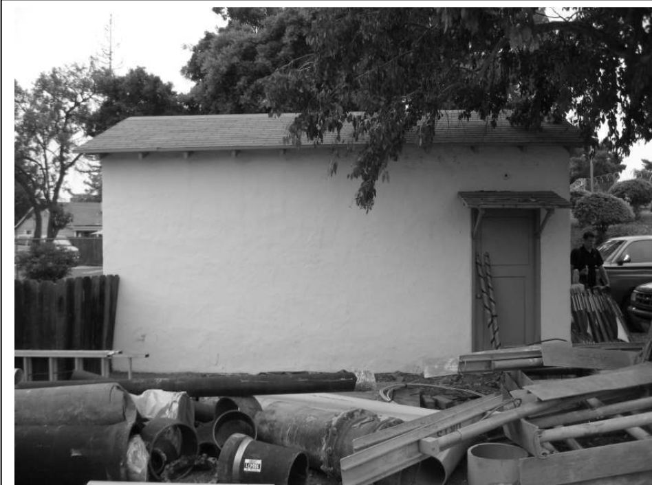
Photo 7: View of the east façade of the Fountain Pump House.
