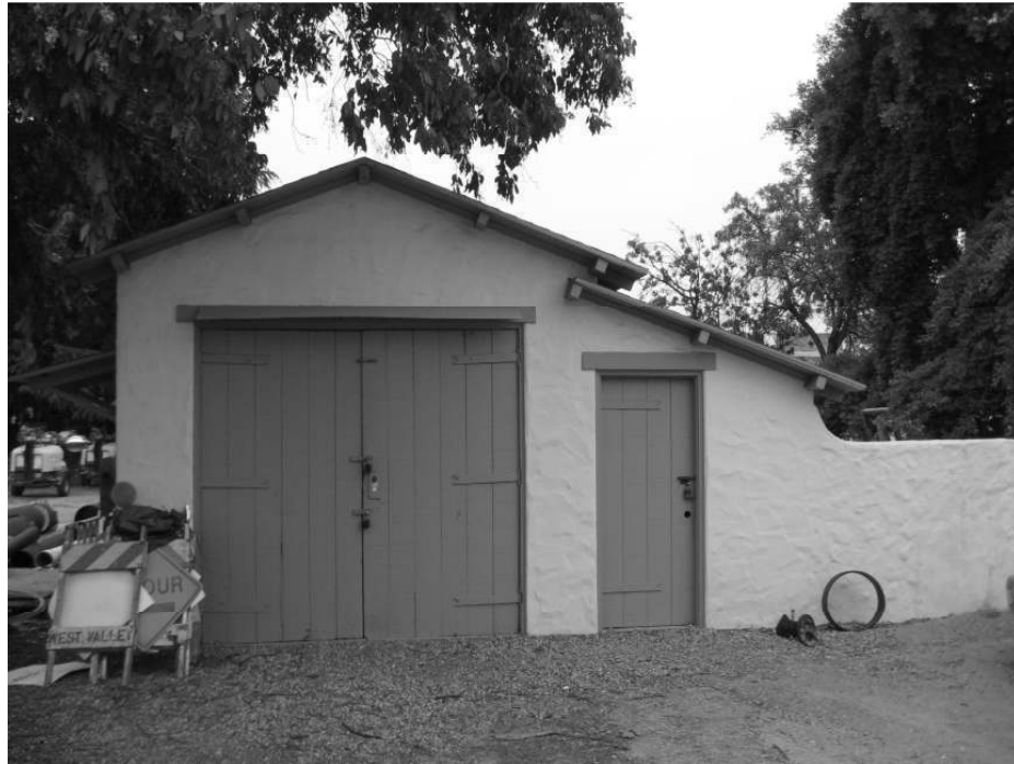
Photo 3: View of the front façade of the Fountain Pump House.
