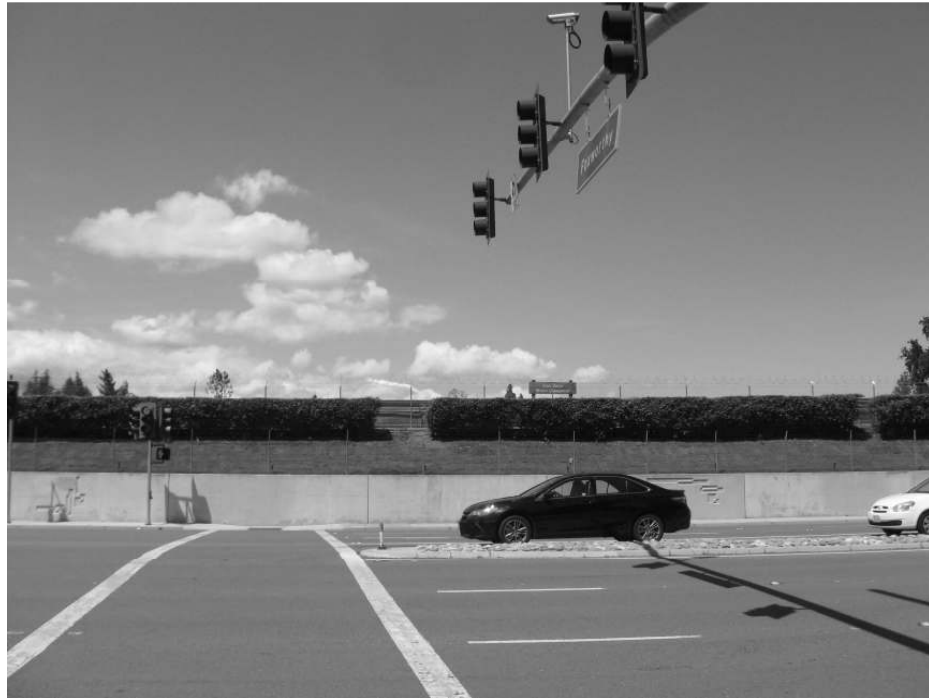
Photo 25: Overview shot of the Cambrian Station from across Bascom.
