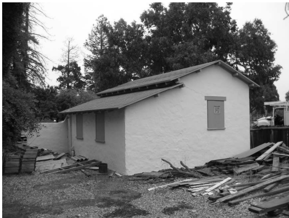
Photo 6: View of the rear façade of the Fountain Pump House.
