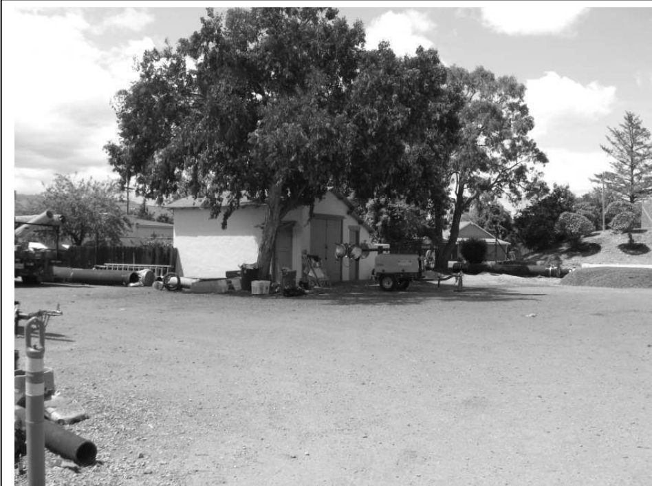
Photo 1: Oblique view of the Fountain Pump House.
