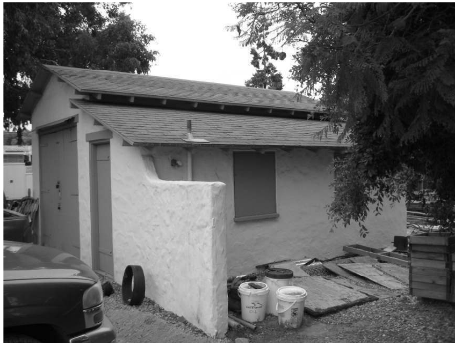
Photo 1: View of the western façade of the Fountain Pump House.
