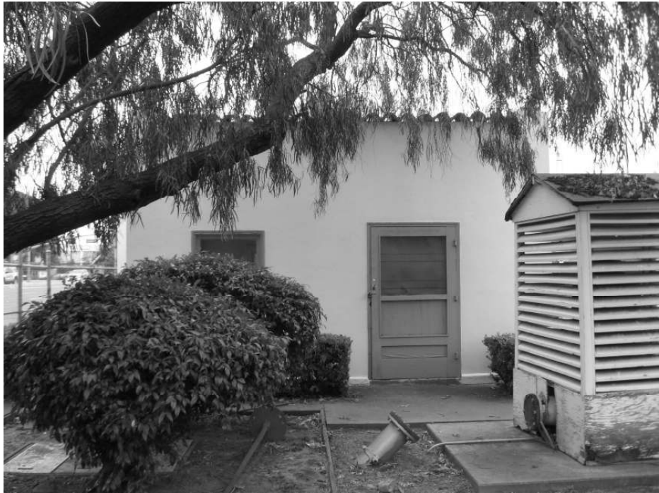
Photo 21: View of the northern façade of the Booster Pump Building.
