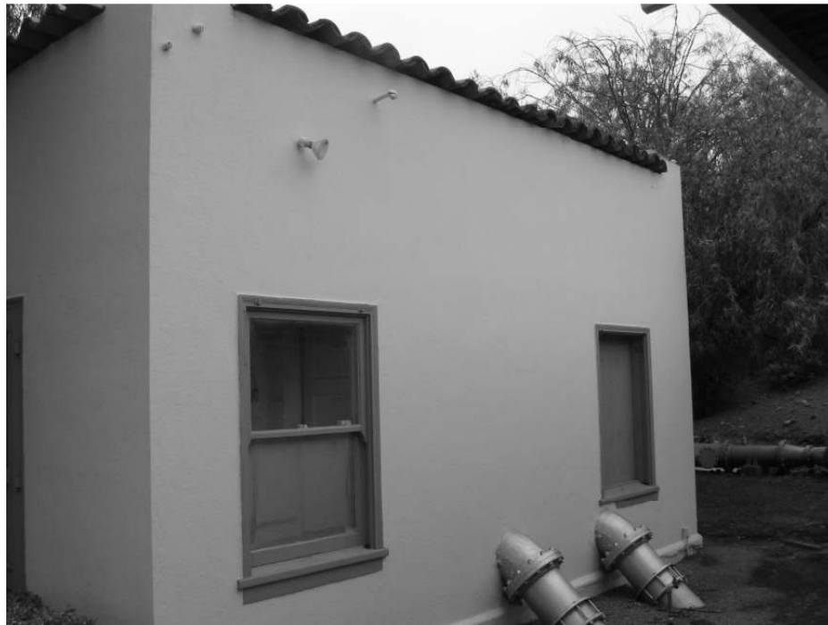
Photo 23: View of the rear façade of the Booster Pump Building.
