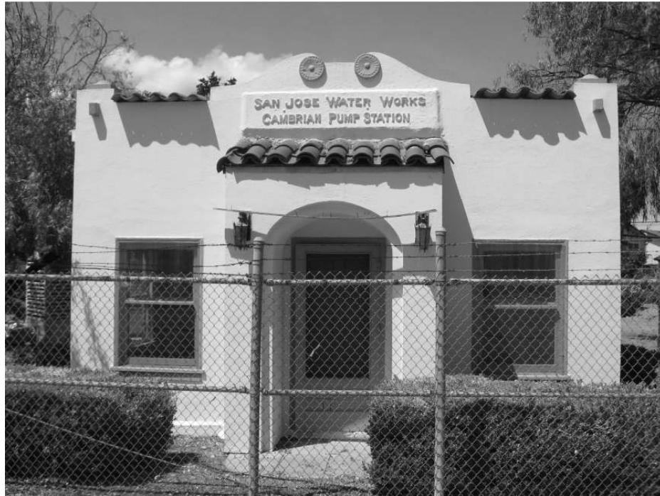
Photo 17: View of the front façade of the Booster Pump Building.
