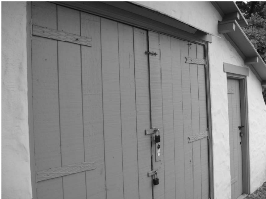
Photo 8: Detail of the large bay door on the Fountain Pump House.
