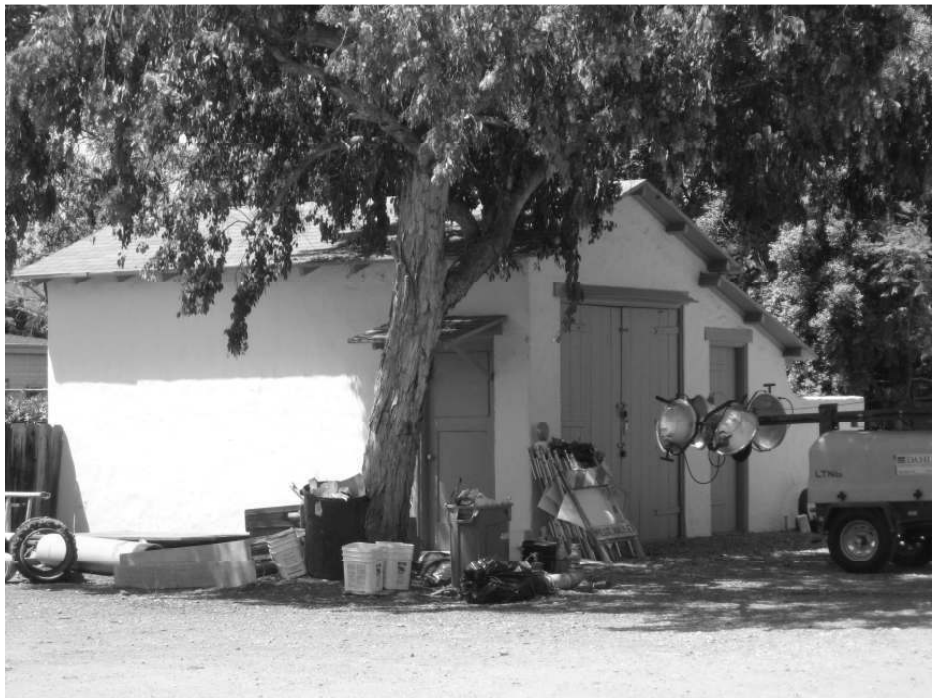
Photo 2: A closer oblique view of the Fountain Pump House.
