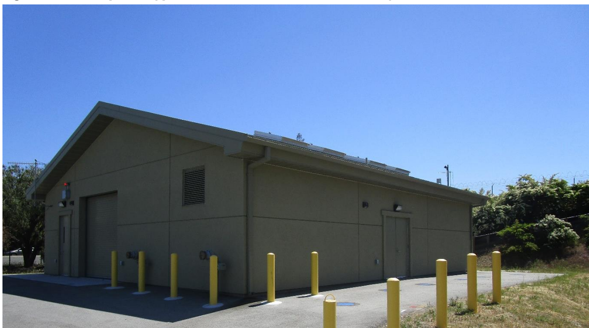
Figure 6 North (Primary) and West Elevations of 2020 Pump House, View Southeast
