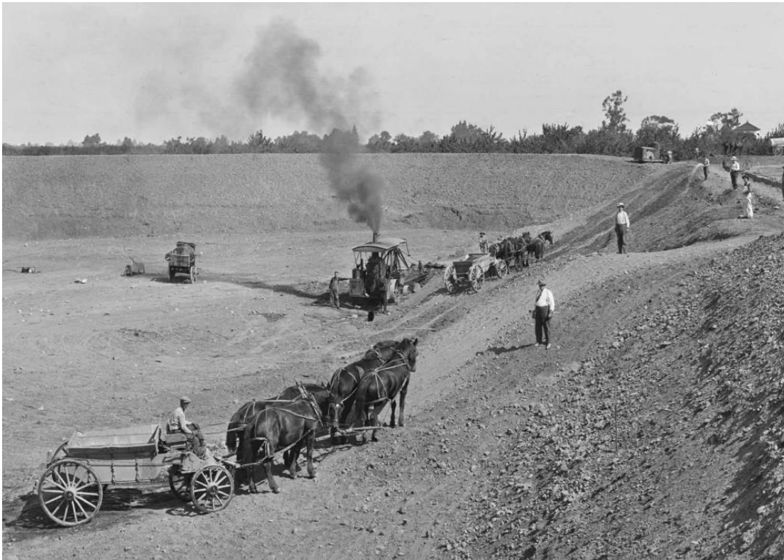
Figure 12 Construction of the 1921 Reservoir, 1890 Reservoir on the Right
