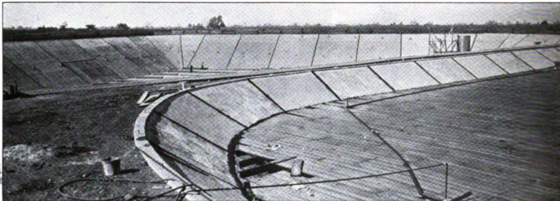
CAMBRIAN RESERVOIRS. NEW RESERVOIR IN BACKGROUND, OLD RESERVOIR IN FOREGROUND DURING RECONSTRUCTION BEFORE OLD ROOF WAS REMOVED
