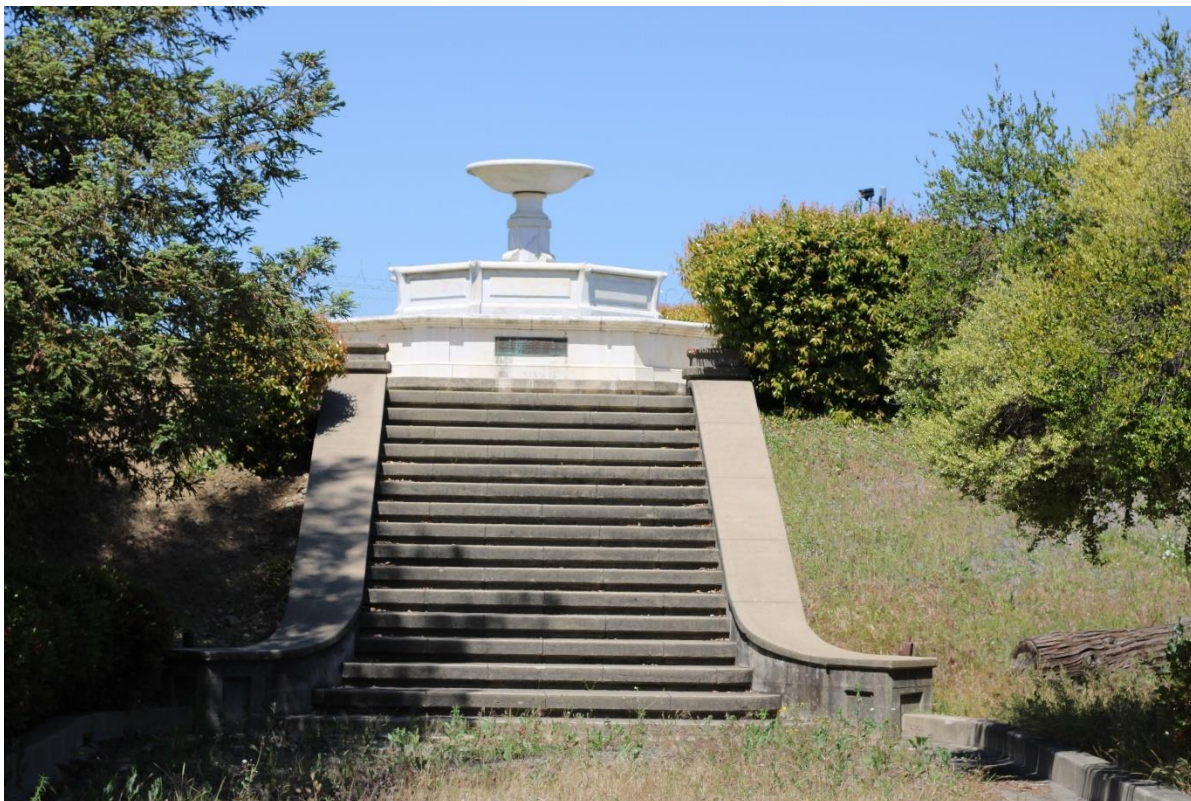
Figure 7 1926 Fountain and Stairs, View North
