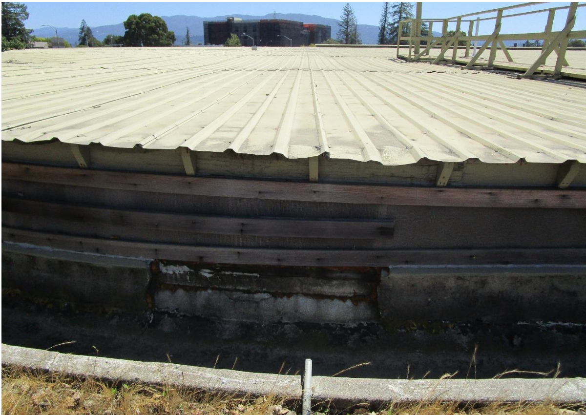
Figure 1 1921 Reservoir, View East
