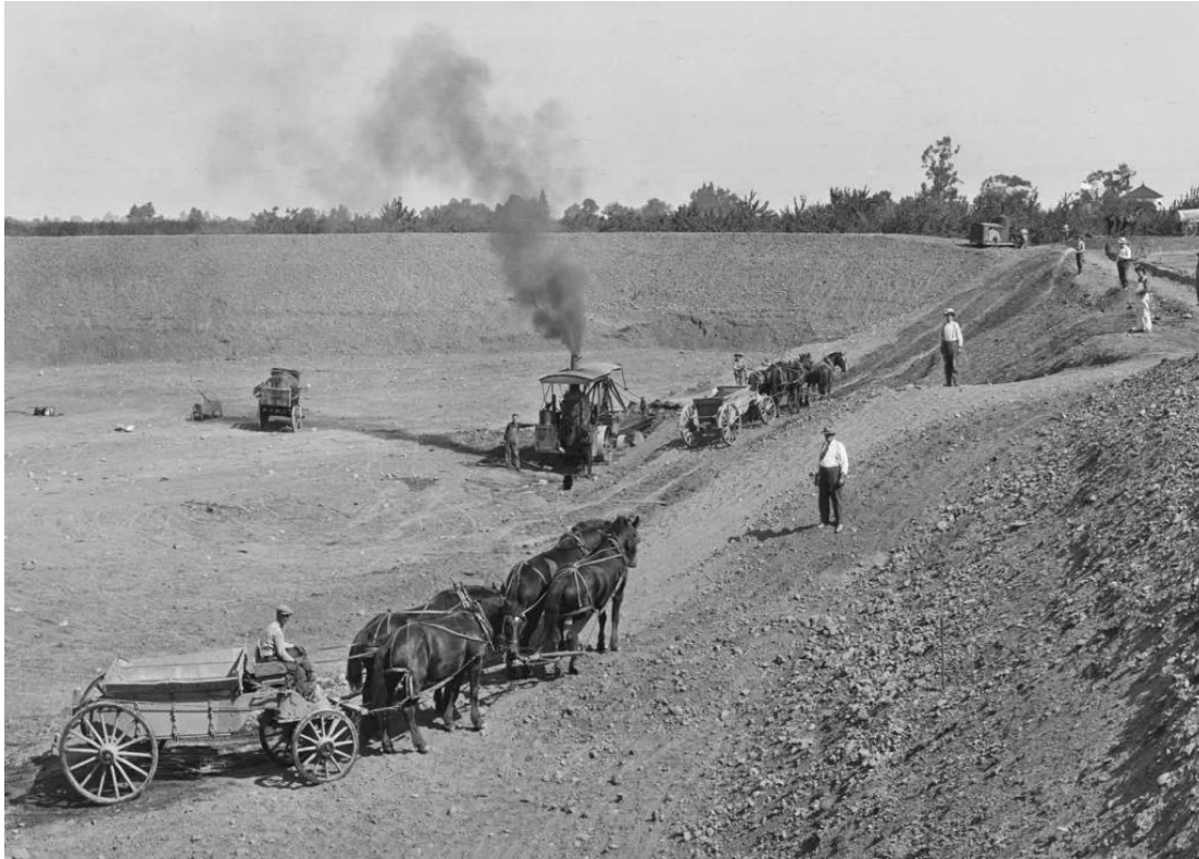
Figure 9 Construction of the 1921 Reservoir, 1890 Reservoir on the Right
