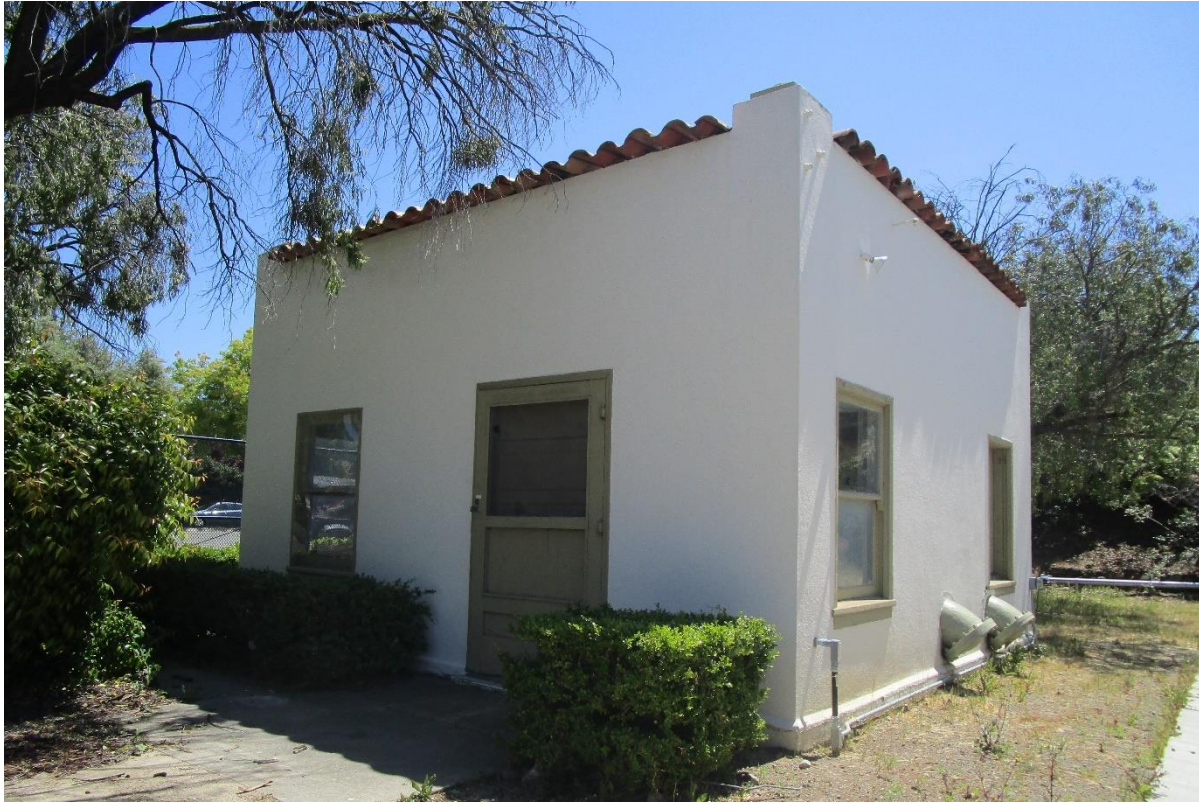
Figure 5 North (L) and West (R) Elevations of 1924 Pump House, View Southeast
