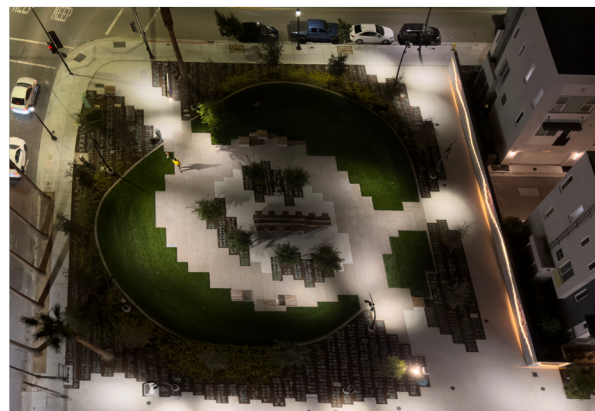
Pellier Park seen from above at night.
