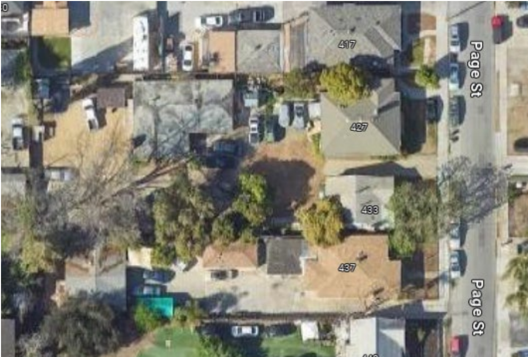
Image 3.1: Aerial View of Property at 427 and 433 Page Street, San Jose, CA
