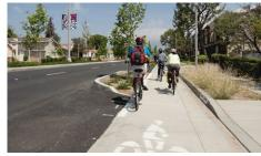
Separated, dedicated bike facilities that provide physical vertical and horizontal separation from motor vehicles
