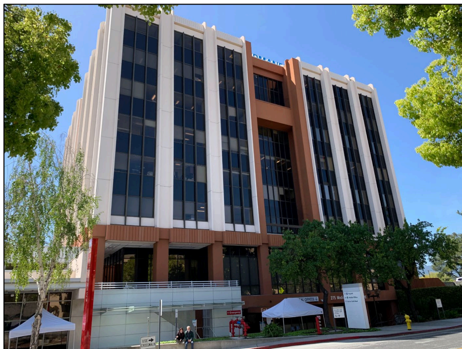
P5b. Description of Photo: 275 Hospital Parkway, facing southwest
