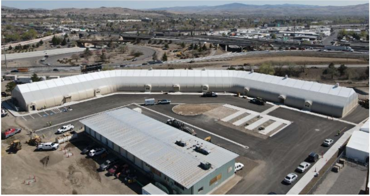
Example 8: Nevada Cares Campus, 1,000 Residents, 60-day Construction
