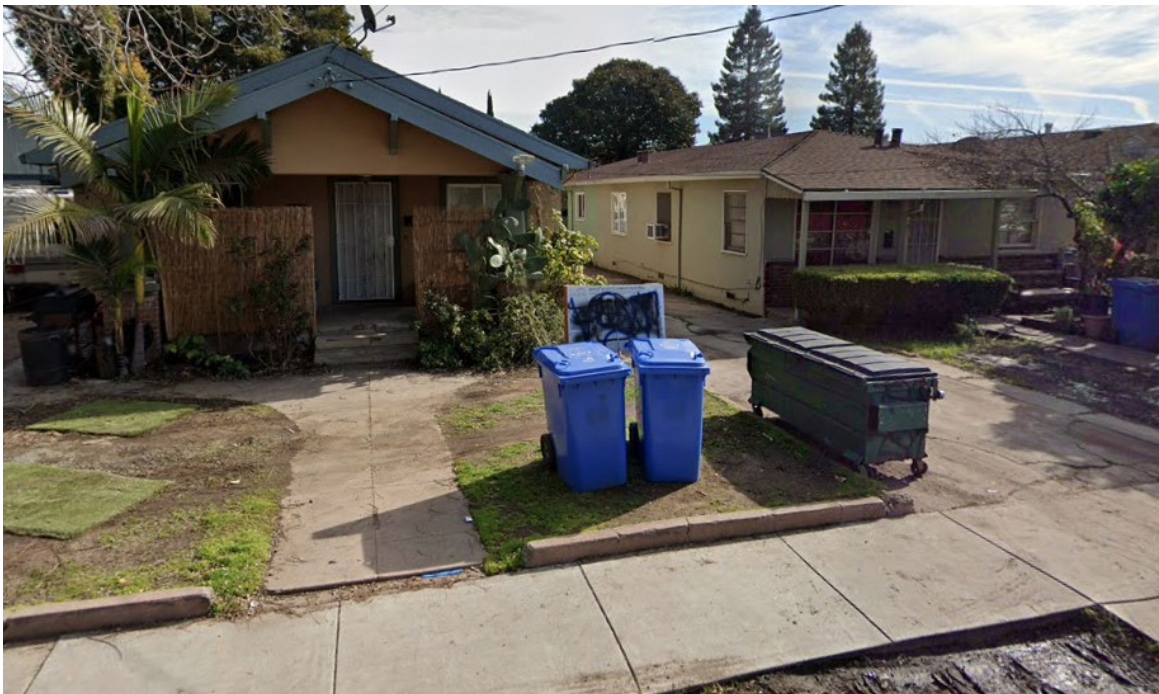
Image 3.2: SFR at 426 (left) and SFR at 430 (right) Page Street, San Jose, CA
