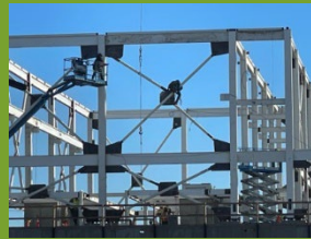
Dewatering Building steel erection
