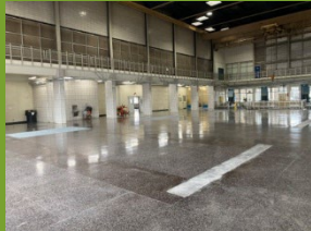
Newly completed terrazzo flooring in Blower Building
