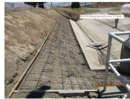
Rebar installation for V-ditch
