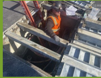
McGrath labeling conduits in handholes
