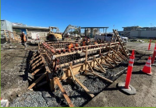
Rebar installation for Fish Screening concrete pad
