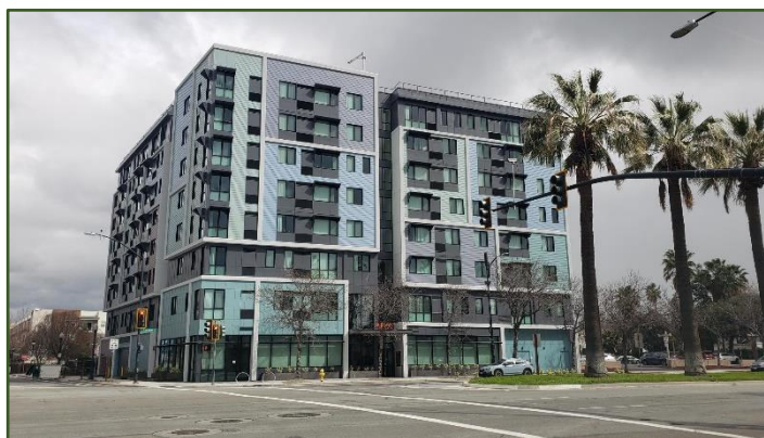
Affordable Housing Project at Balbach & Almaden Blvd
