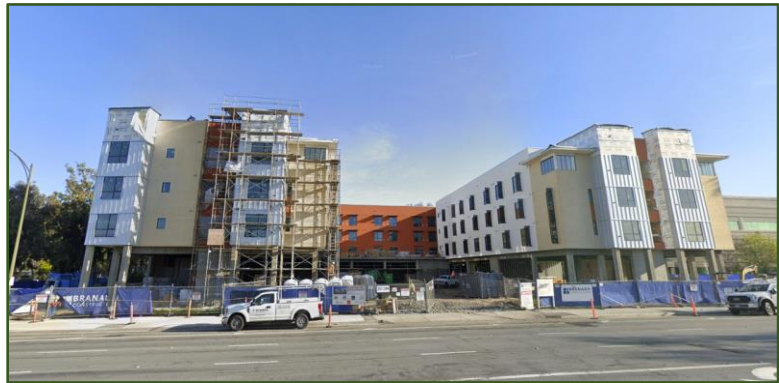
Affordable Housing 397 Blossom Hill Road (Under Construction)
