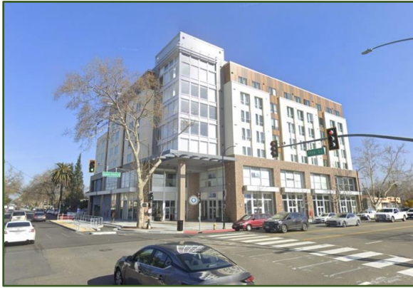
Sparta Student Housing (Construction Complete in 2022)
