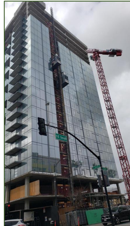
10 East Reed Street Residential Development Under Construction
