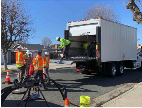
Sanitary Sewer Repairs Project (CIPP Liner Installation)
