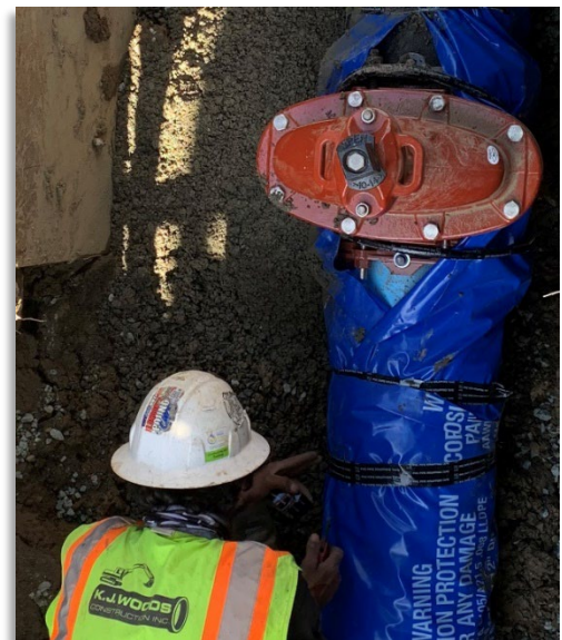
Installation of a water valve
