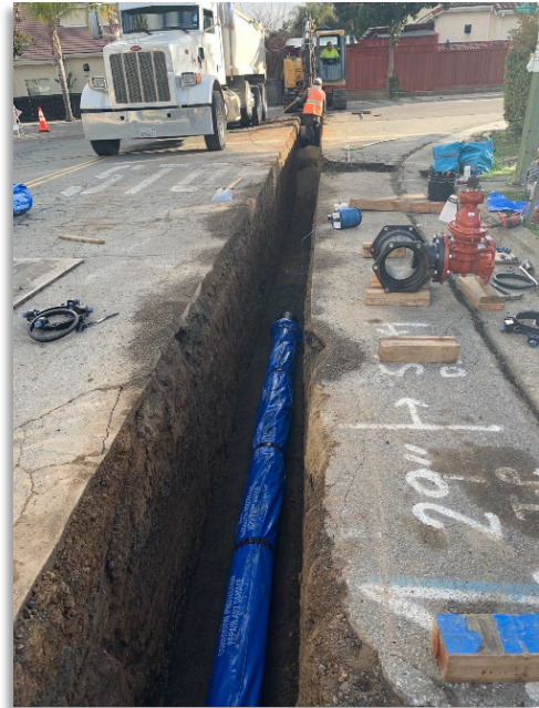
Preparing for a water main installation
