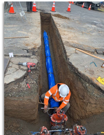
Construction of a main replacement project
