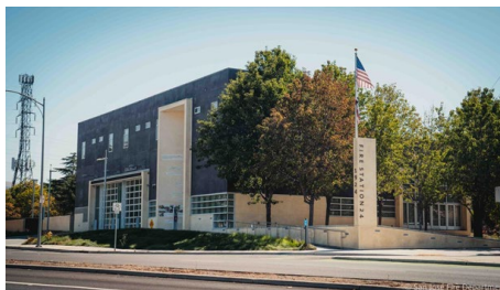
Fire Station 24 Remediation – Completion of Unfinished Rooms
