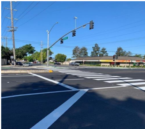
High visibility crosswalk at Senter Road and Umbarger Road
