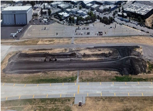
Taxiway V Reconstruction - Phase 1A
