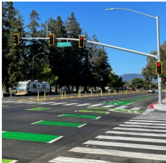
Hillsdale Ave (Almaden Ex to Ross Ave) – lane reduction, bike lanes, quick-build median island and high visibility crosswalks
