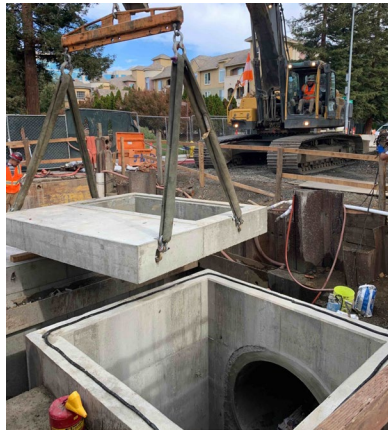
Top of Precast PCC Vault
