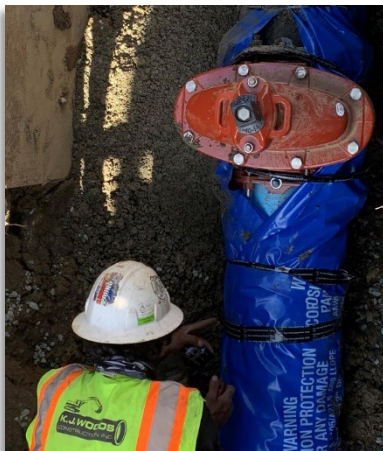
Installation of a water valve
