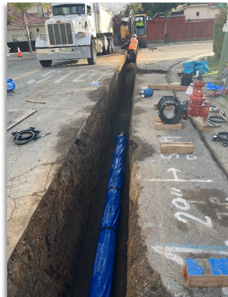
Municipal Water Main Construction Work
