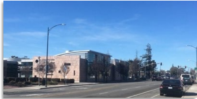
Undergrounding - Dr. Robert Cruz Alum Rock Branch Library West side of White Road, south of Alum Rock Avenue
