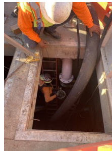
Contractors carry out wet well rehab work
