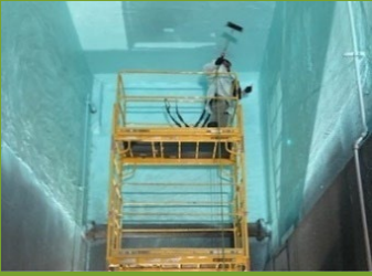
Installing epoxy inside No. 3 Water Wet Well
