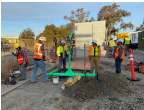
Electrical vault drain installation
