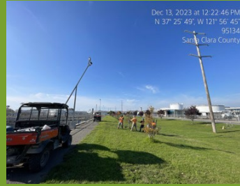
Contractors Overaa and McGrath changing a light ballast at Basin B1
