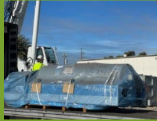
Centrifuge #1 arriving at the jobsite
