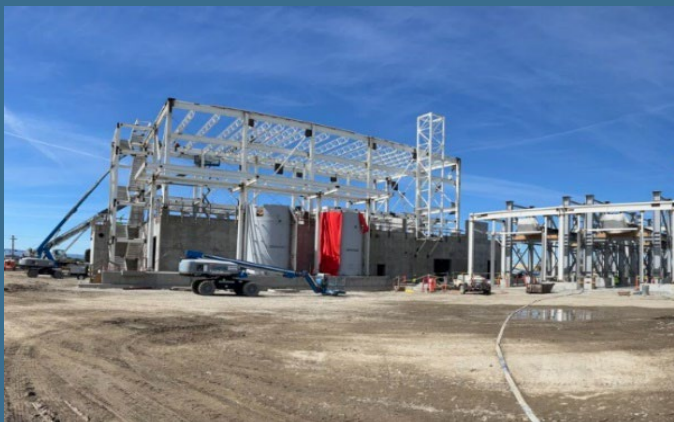
Construction underway at the Dewatering and Truck Loadout Buildings taken March 2024
