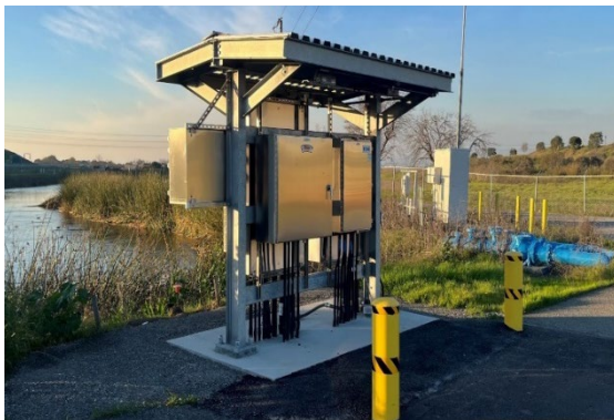
Daylight Station with newly installed panels and canopy
