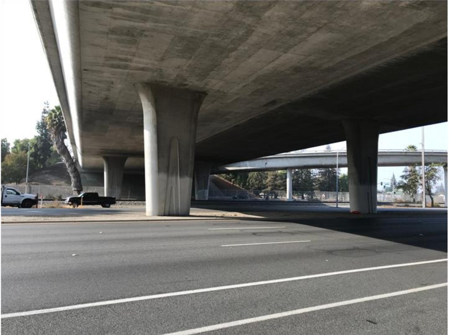
Photo 4: The Blossom Hill overcrossing bridge support columns.
