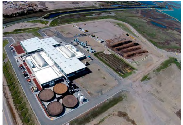
Zero Waste Energy Development Company Organics Processing Facility
