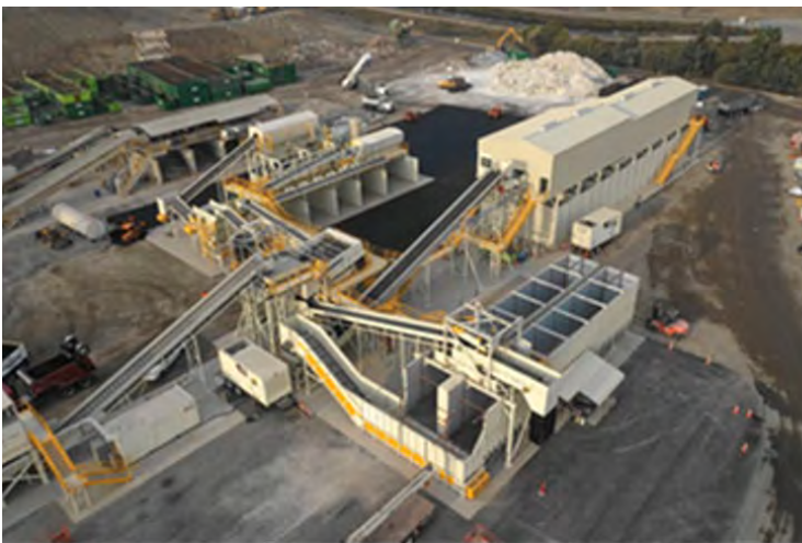
Zanker Recycling Construction Debris Processing
