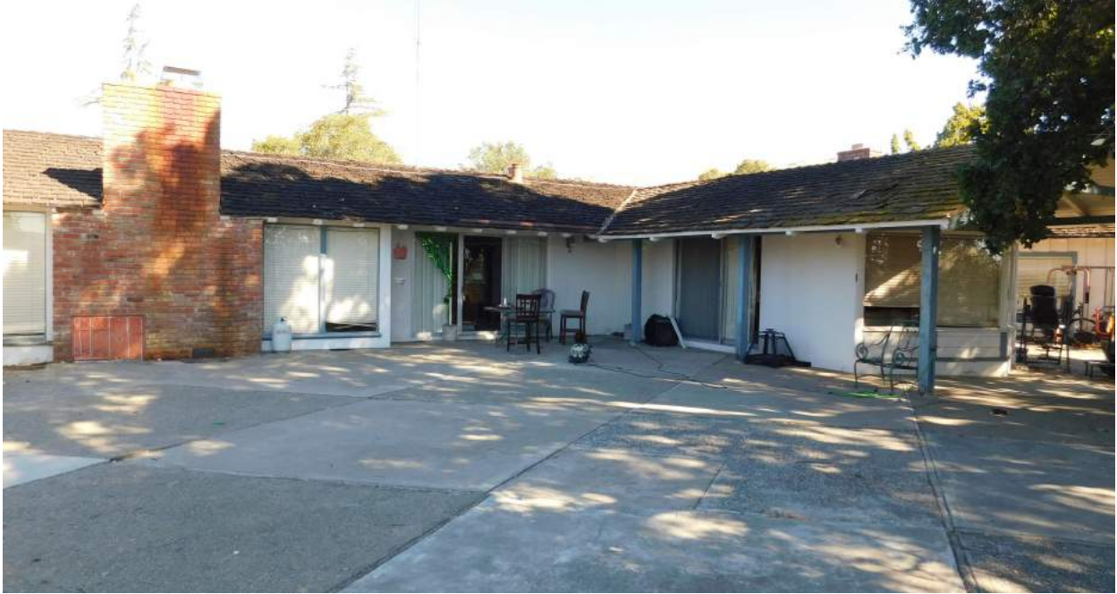
Rear southwest back yard
