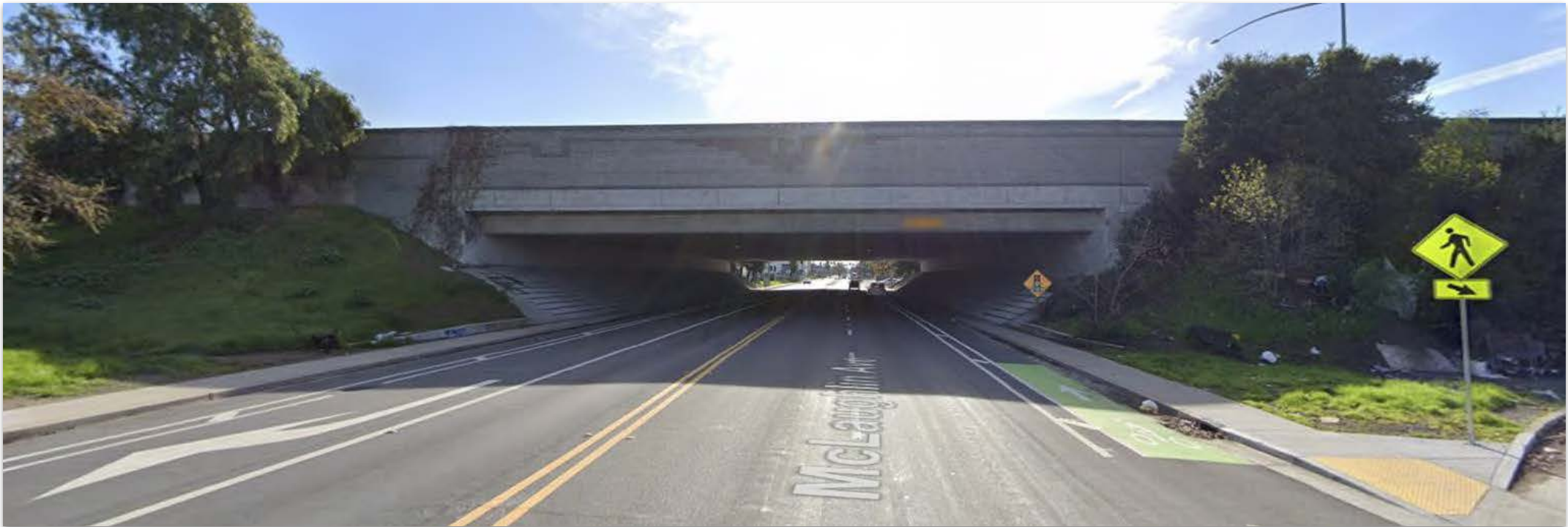
I-280 & McLaughlin Ave Overpass Source: Google Maps
