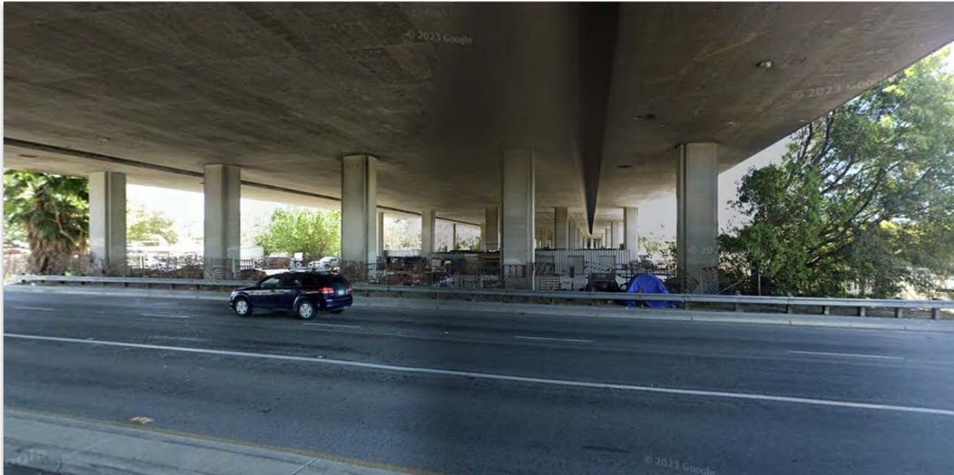
Parking/storage area under the highway Source: Google Maps
