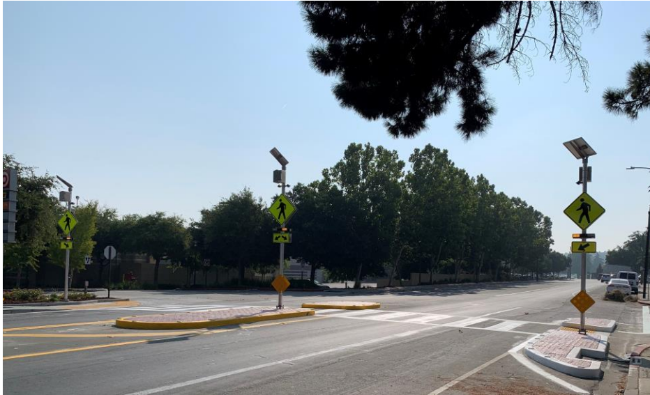
Enhanced Crosswalk with RRFBs Little Orchard / Perrymont
