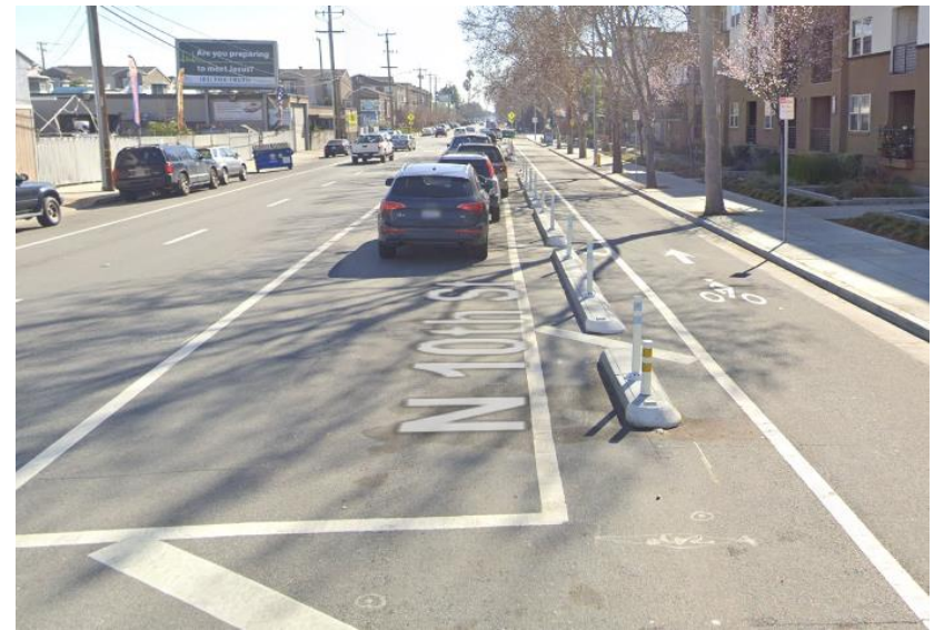
Example of concrete separated bike lanes
