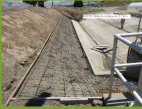
V-ditch rebar installation
