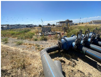
Santa Clara influent control structure
