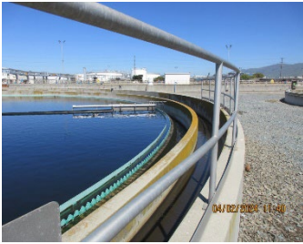
B7 Clarifier baffle reset
