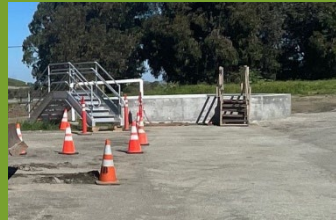
Fish screen with newly added perimeter containment wall and grate
