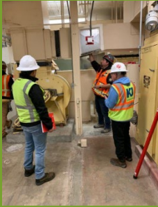
Installing Admin Building duct detectors
