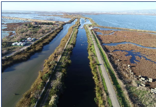
Outfall Channel discharging treated wastewater into the South Bay
