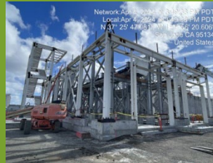
Truck load-out building structural steel
