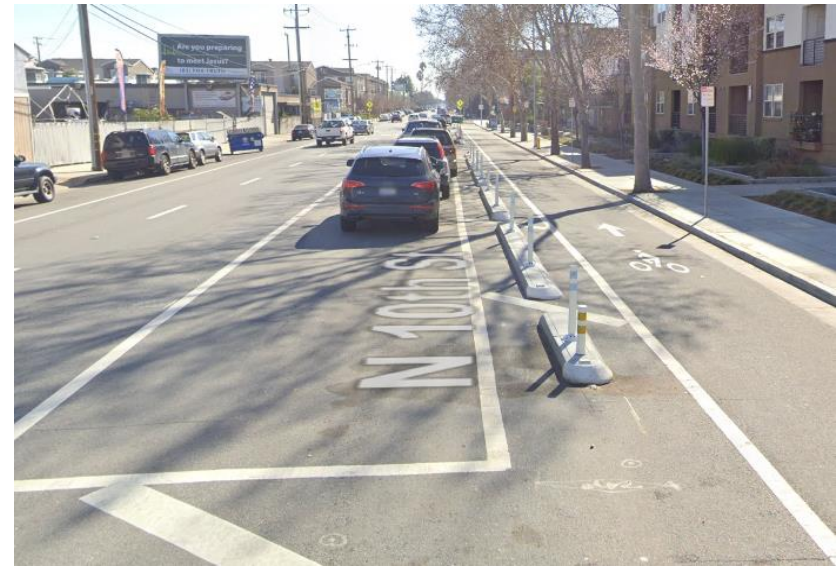
Example of concrete separated bike lanes
