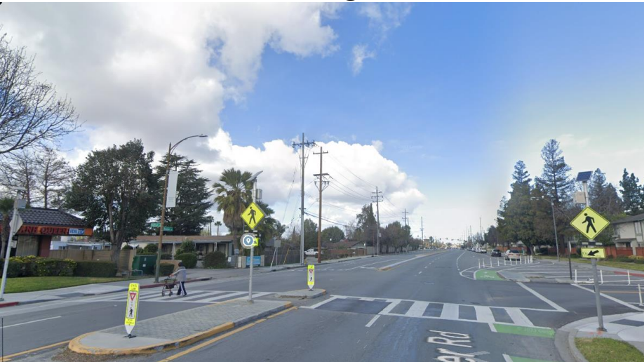
Flashing beacon (Installed in 2013)
