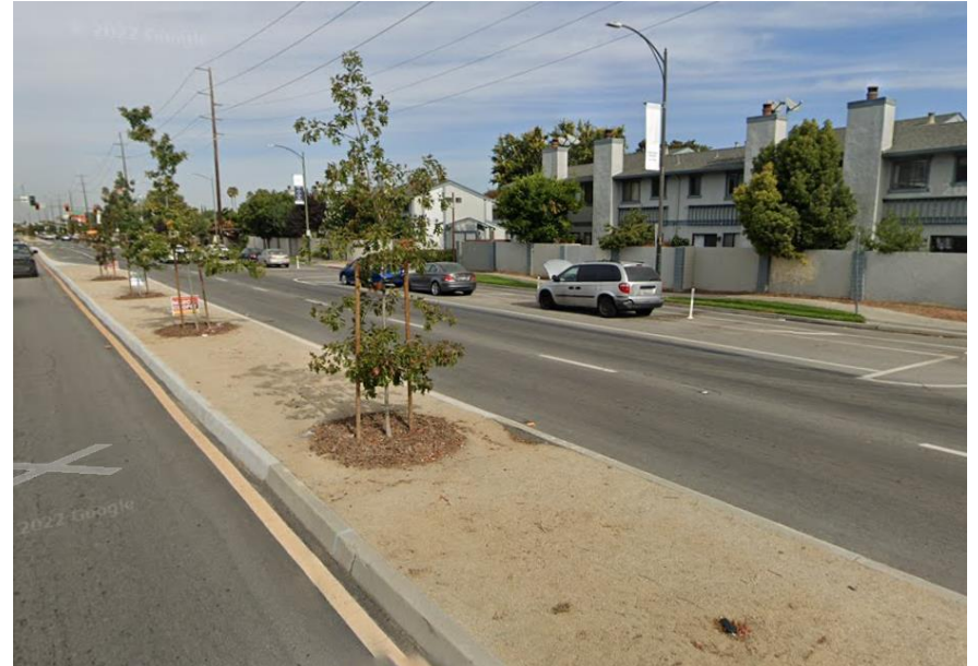
Median Extension & Additional Trees: Senter & Umbarger (AFTER)
