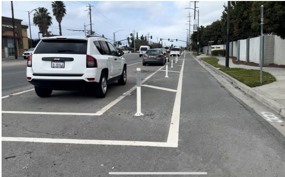
Existing quick-build vertical delineators on Senter
