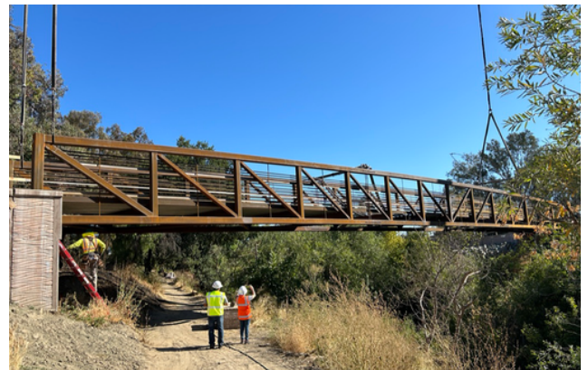
Coyote Creek Trail pedestrian bridge installation
