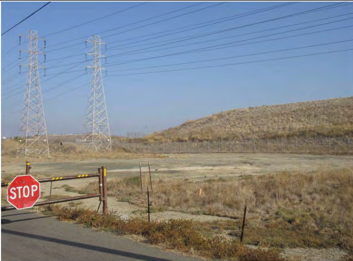
Photo 5 Looking east toward the NW Basin site from the entrance gate of the Don Edwards National Wildlife Refuge on Grand Boulevard.
