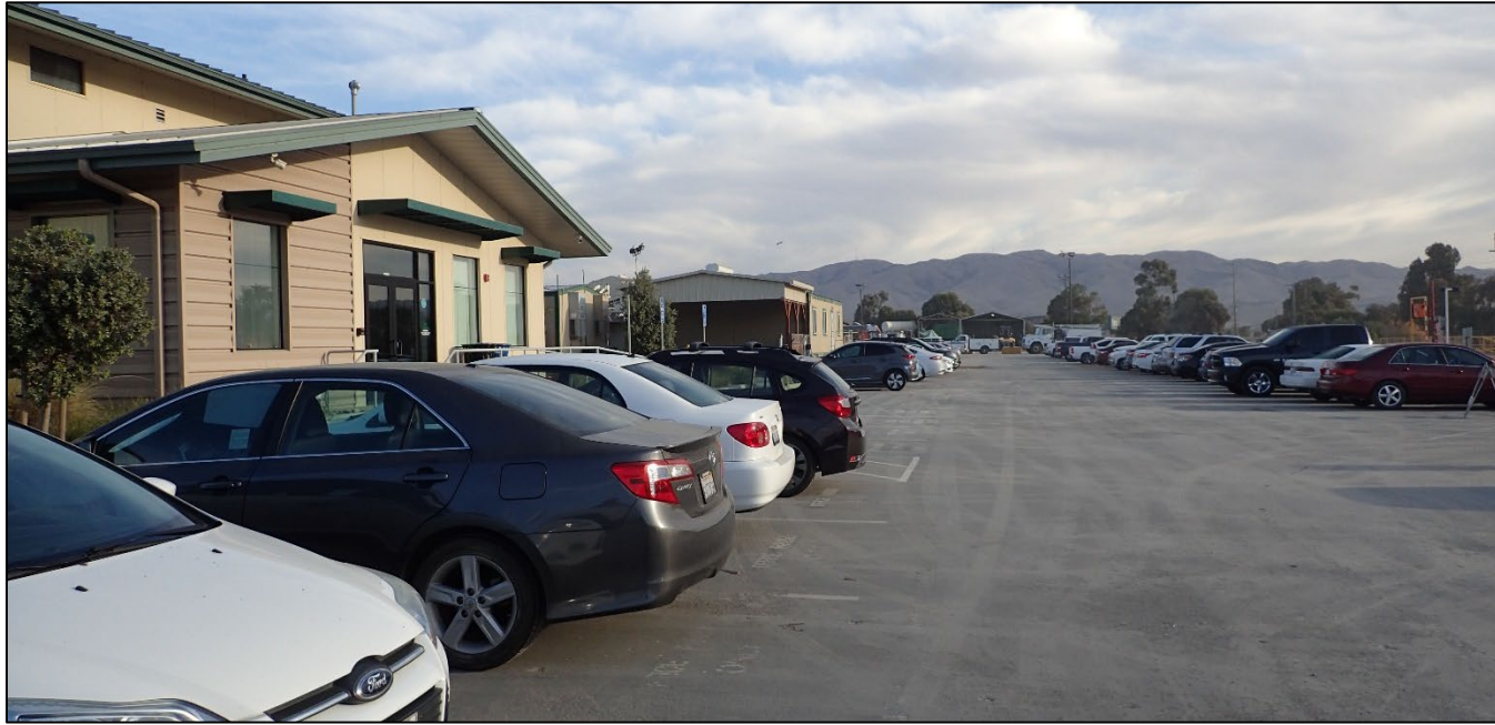
Photograph 1. Photo of developed hardscape in the southwest corner of the WMU, facing northeast. Photo taken in the office parking lot.
