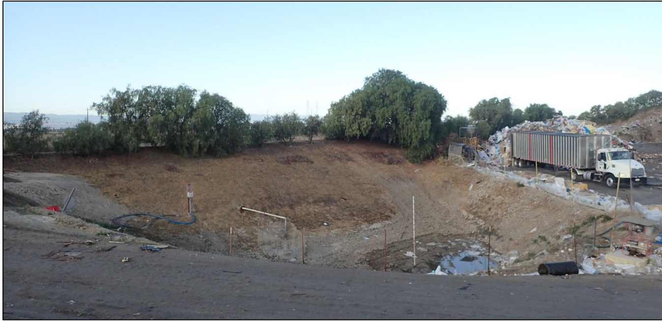
Photograph 5. Photo of a wastewater pond located in the southwest part of the WMU, facing west. A row of planted ornamental Peruvian peppertrees can be seen in the background.
