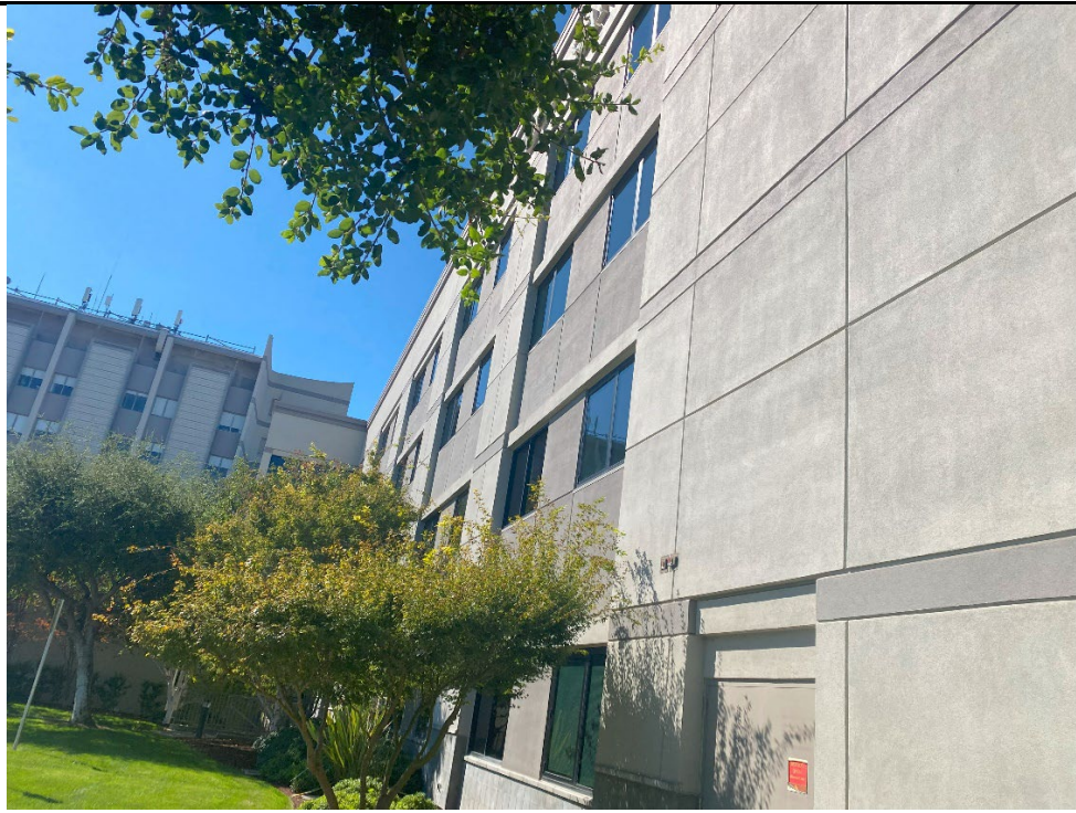
8. This photo depicts one of the hospital building's exterior walls.
