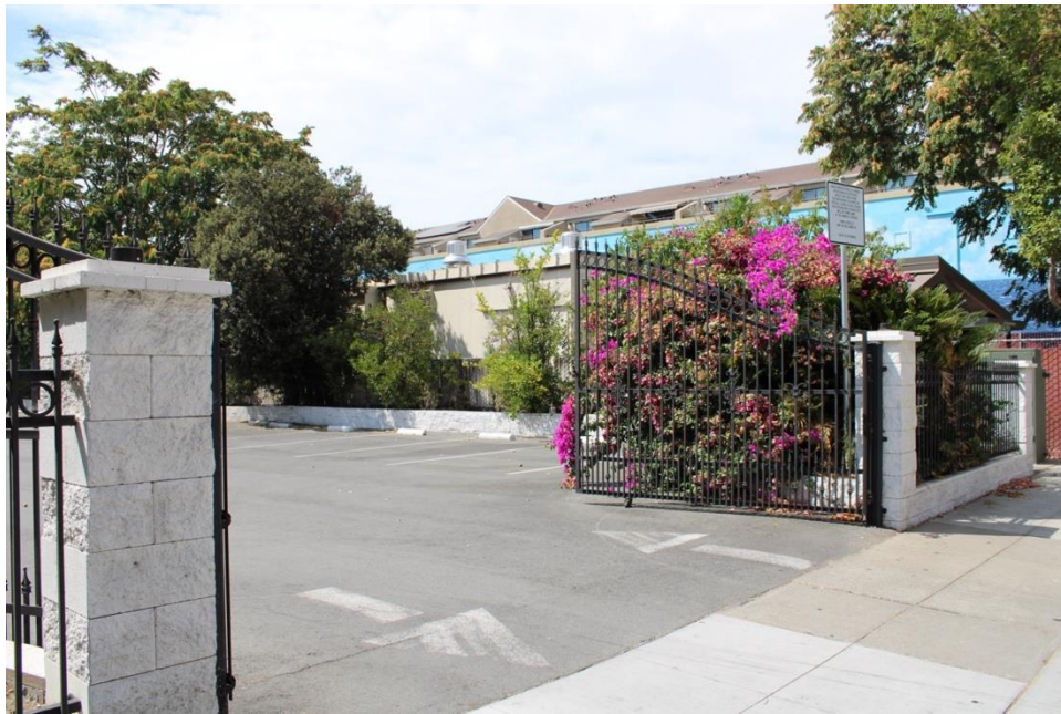
Figure 33. Automatic double gate, providing access to paved parking lot, facing north.
