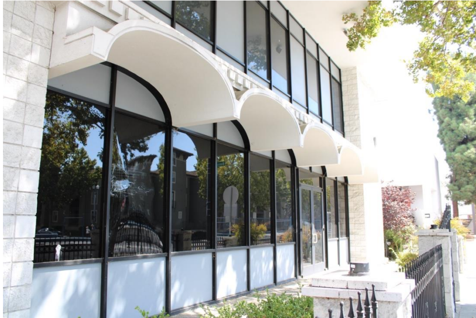
Figure 6. Decorative belt course and metal arched hood.
