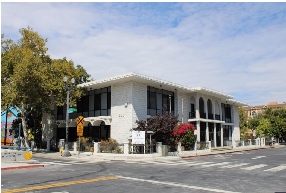
Figure 19. Southwest and southeast elevations, facing north.
