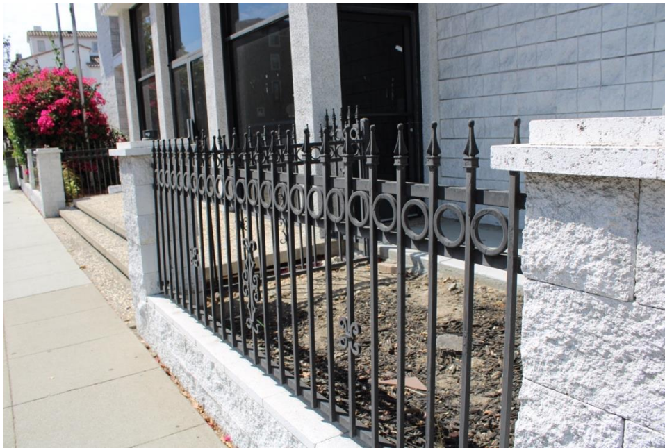
Figure 12. Wrought-iron fence, with concrete block posts.
