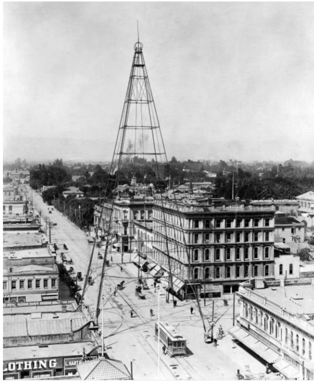
Figure 8. 1910 photograph of the San Jose Electric Light Tower and interurban rail line that ran north-south through the center of downtown along 1 st Street (courtesy of the San Jose Public Library).
