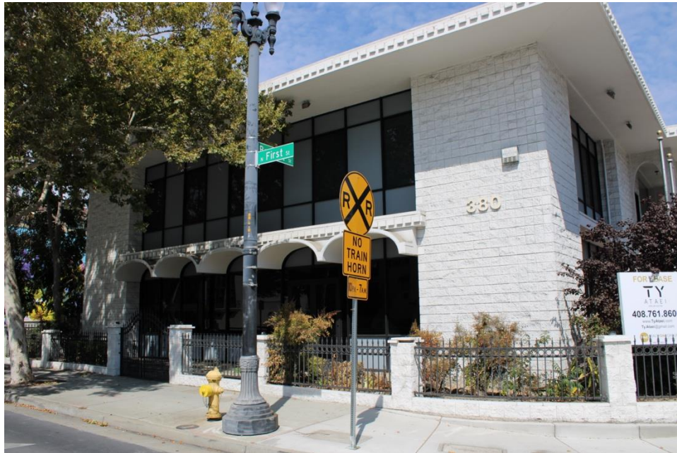
Figure 5. Southwest elevation, facing north.
