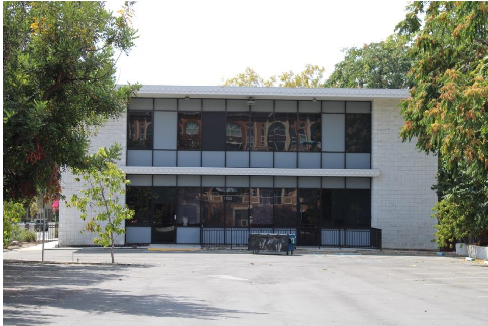
Figure 10. Northeast elevation, facing southwest.
