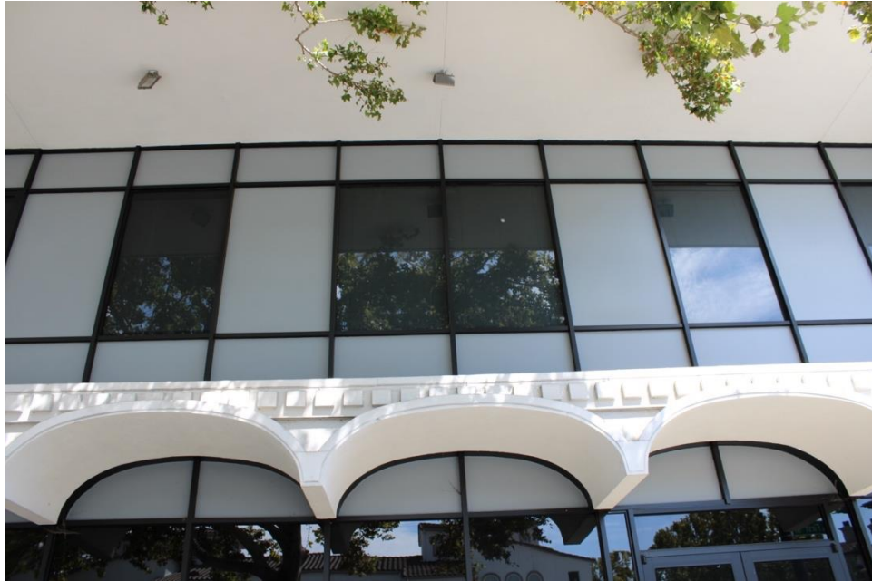
Figure 26. Metal arched hood and frosted glazing.
