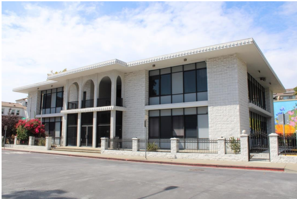
Figure 20. Southeast elevation, facing northwest.
