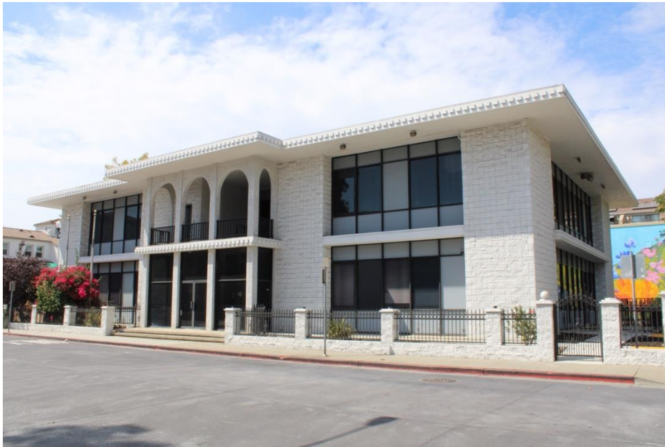
Figure 1. Southeast elevation, facing northwest.
