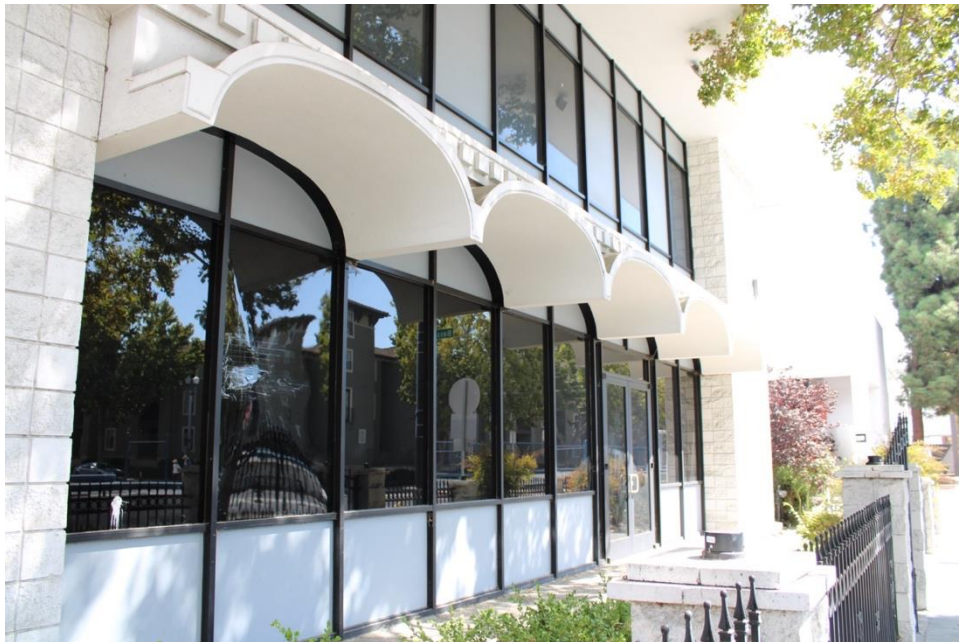
Figure 25. Decorative belt course and metal arched hood.
