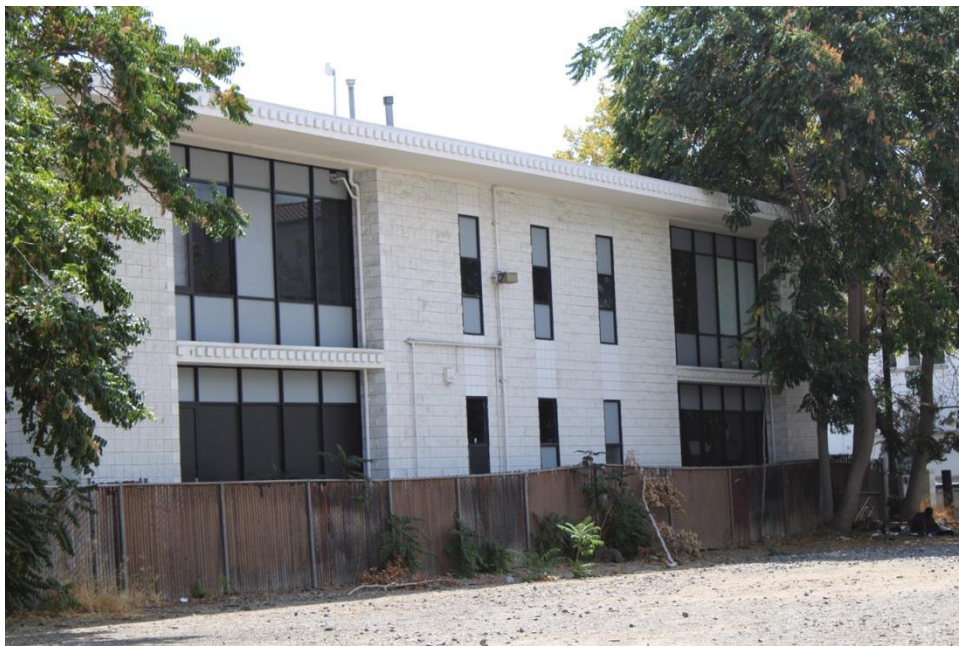
Figure 28. Northwest elevation, facing west.
