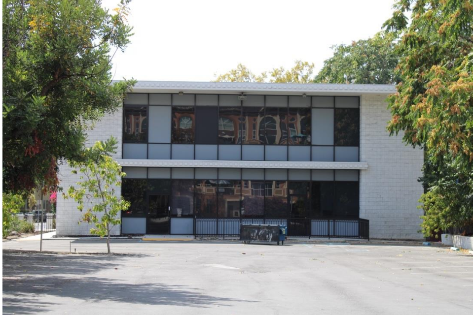
Figure 29. Northeast elevation, facing southwest.
