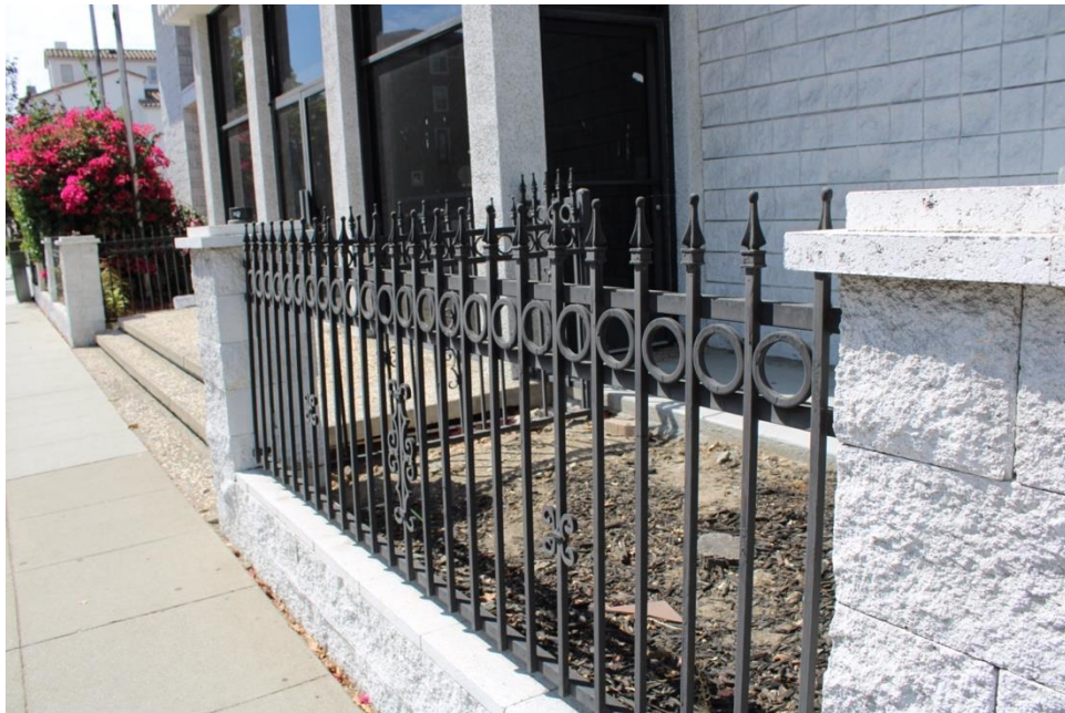
Figure 31. Wrought-iron fence, with concrete block posts.
