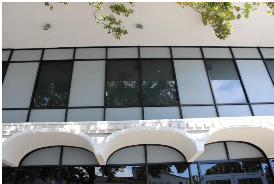
Figure 7. Metal arched hood and frosted glazing.
