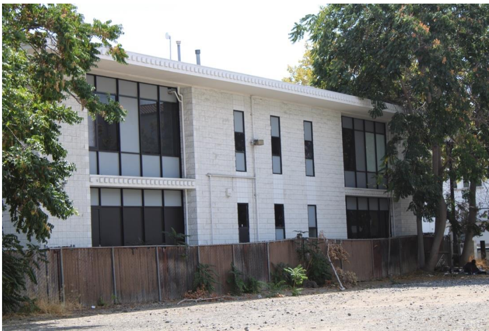
Figure 9. Northwest elevation, facing west.
