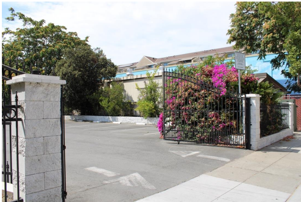
Figure 14. Automatic double gate, providing access to paved parking lot, facing north.
