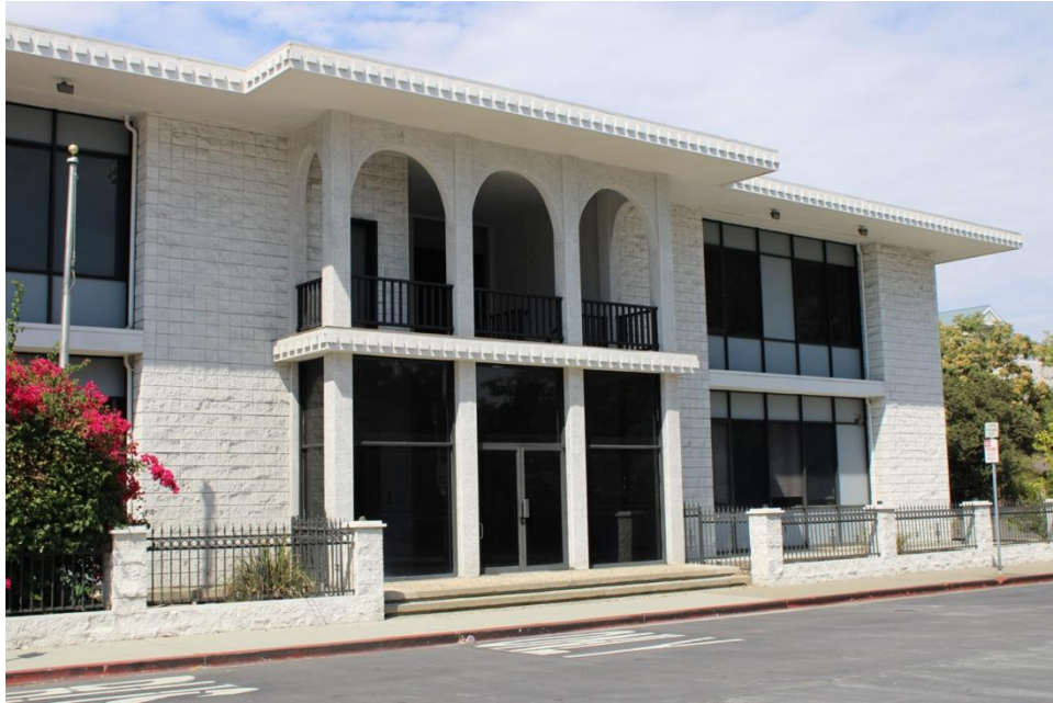
Figure 21. Central, projecting section of southeast elevation, facing northeast.
