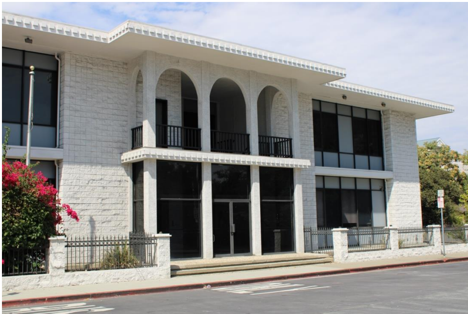
Figure 2. Central, projecting section of southeast elevation, facing northeast.
