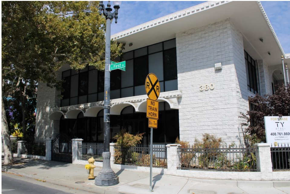
Figure 24. Southwest elevation, facing north.
