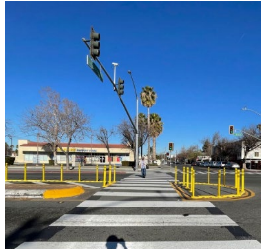
High Visibility Crosswalk – Story Rd (Knox Ave to White Rd)
