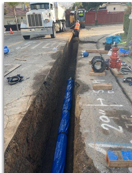
Municipal Water Main Construction Work
