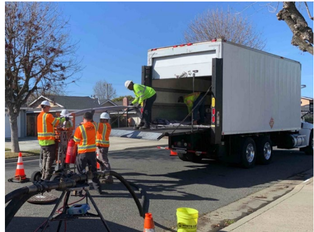
Sanitary Sewer Maintenance Crew
