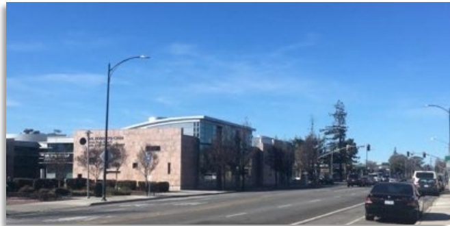
Undergrounding - Dr. Robert Cruz Alum Rock Branch Library West side of White Road, south of Alum Rock
