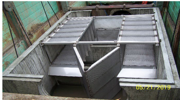
Large Trash Capture device installation near Coyote Creek
