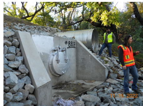
An outfall at Coyote Creek rehabilitated in October 2022
