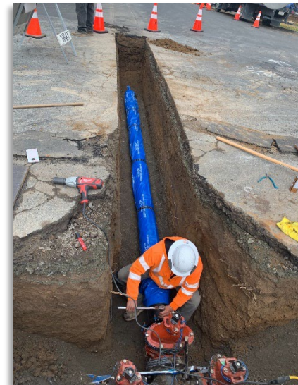
Construction of a main replacement project
