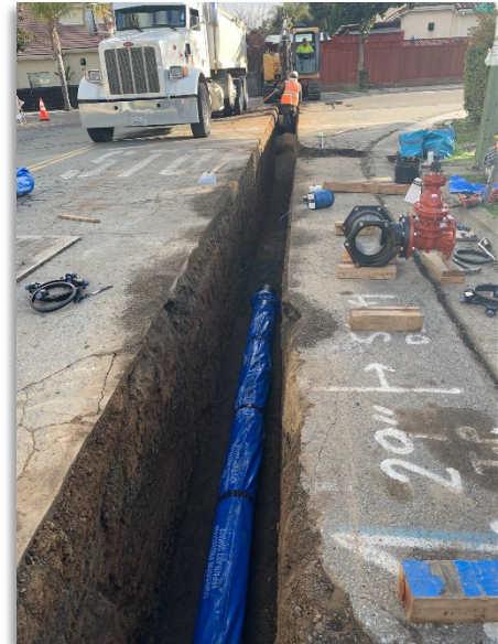
Preparing for a water main installation
