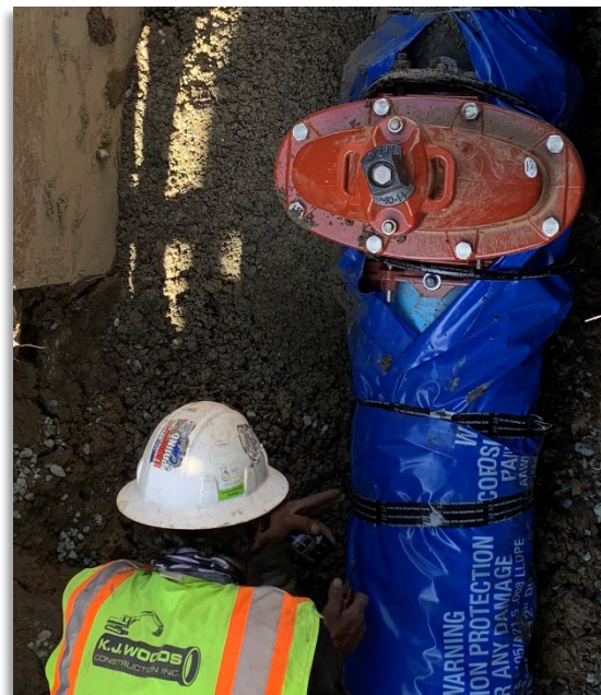
Installation of a water valve
