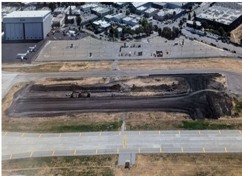
Taxiway V Reconstruction - Phase 1A
