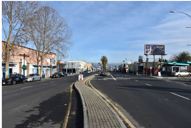
Figure 6: W San Carlos Street looking east.
