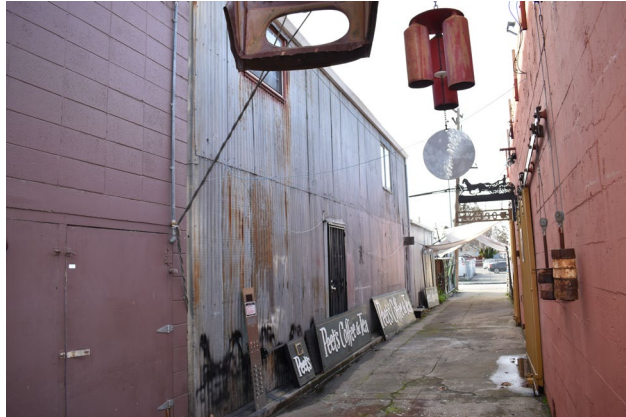
Figure 6. Oblique view of the rear north façade, looking west.
