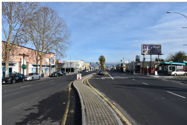
Figure 8: W San Carlos Street looking east.
