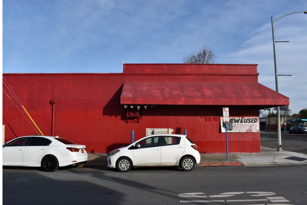
Figure 3. West façade, view east.
