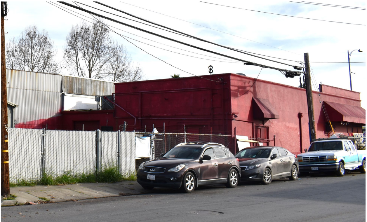
Figure 5: Oblique view of the rear north façade, looking southeast.
