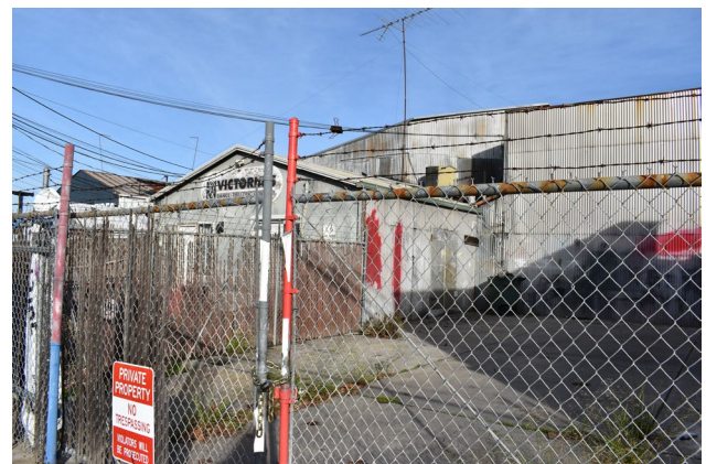
Figure 5. South facade, view northeast.
