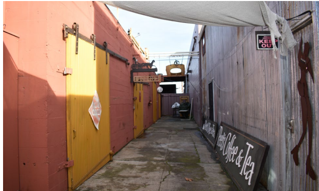
Figure 3: South façade, looking west.
