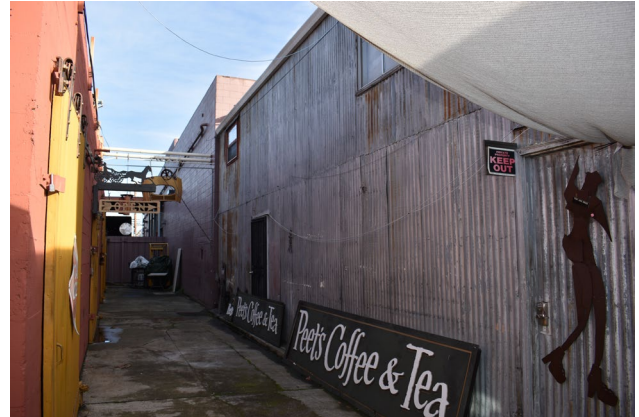
Figure 7. Rear north façade, looking east.
