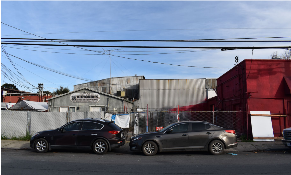
Figure 3: West façade, looking east.
