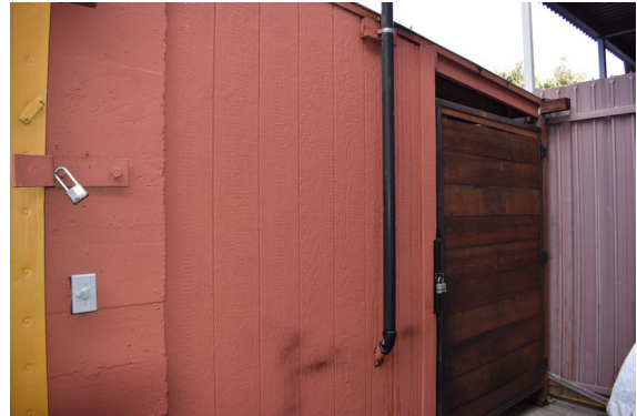
Figure 4: Rear woodshed, looking northeast.
