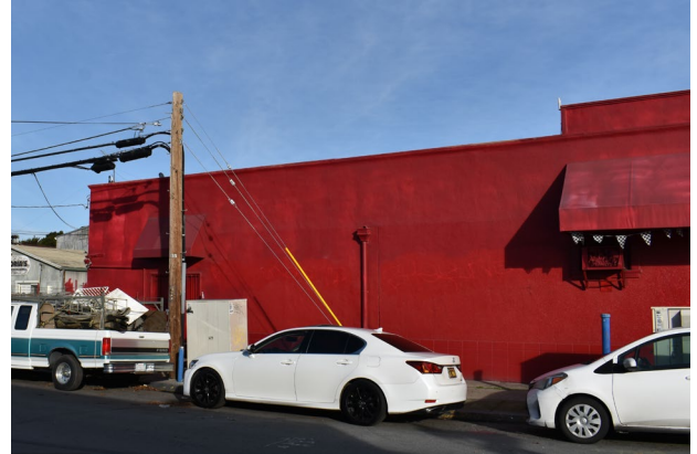
Figure 4. West façade, view northeast.
