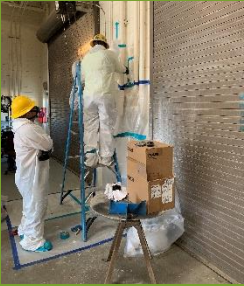
Installing warehouse infrastructure
