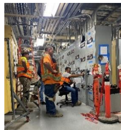
Electrical load migration in progress
