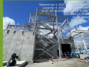
Dewatering Building south stairs
