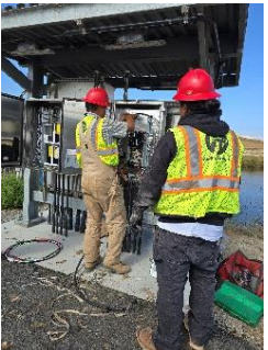
Installing Daylight Station electrical components
