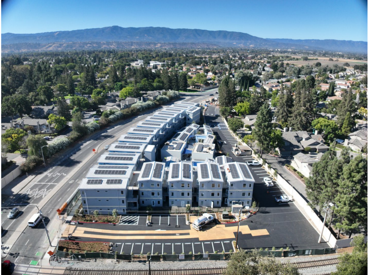
Exterior Side View from Monterey Road
