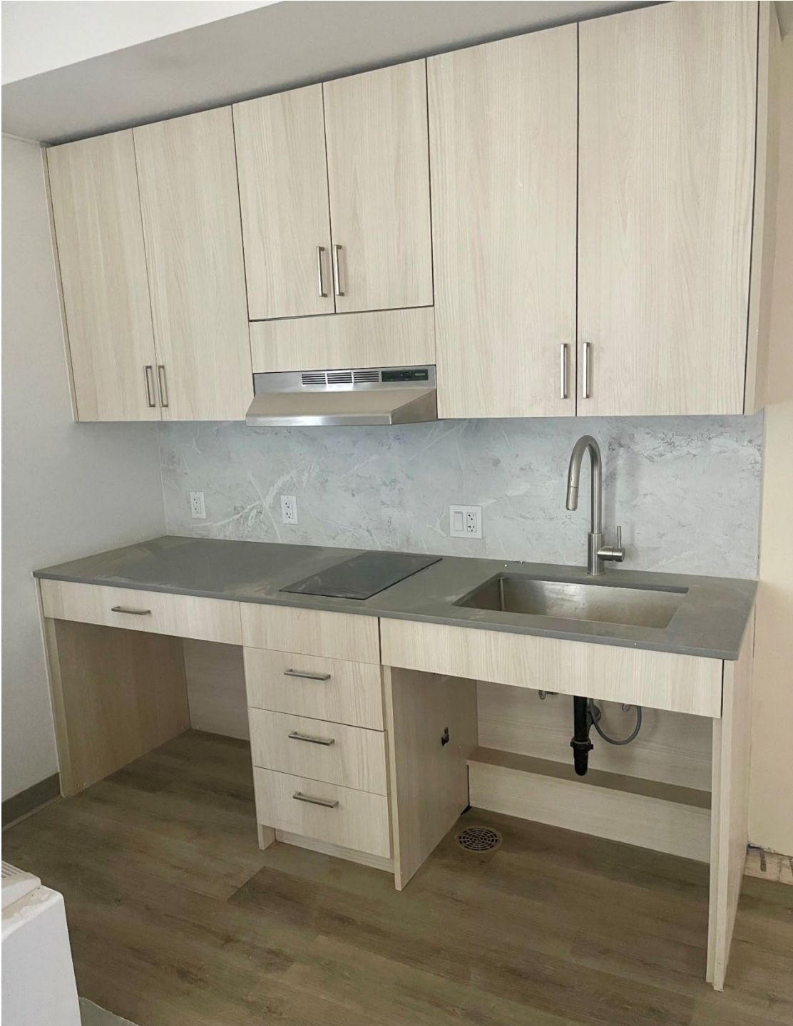
View of Kitchnette within Modular Unit
