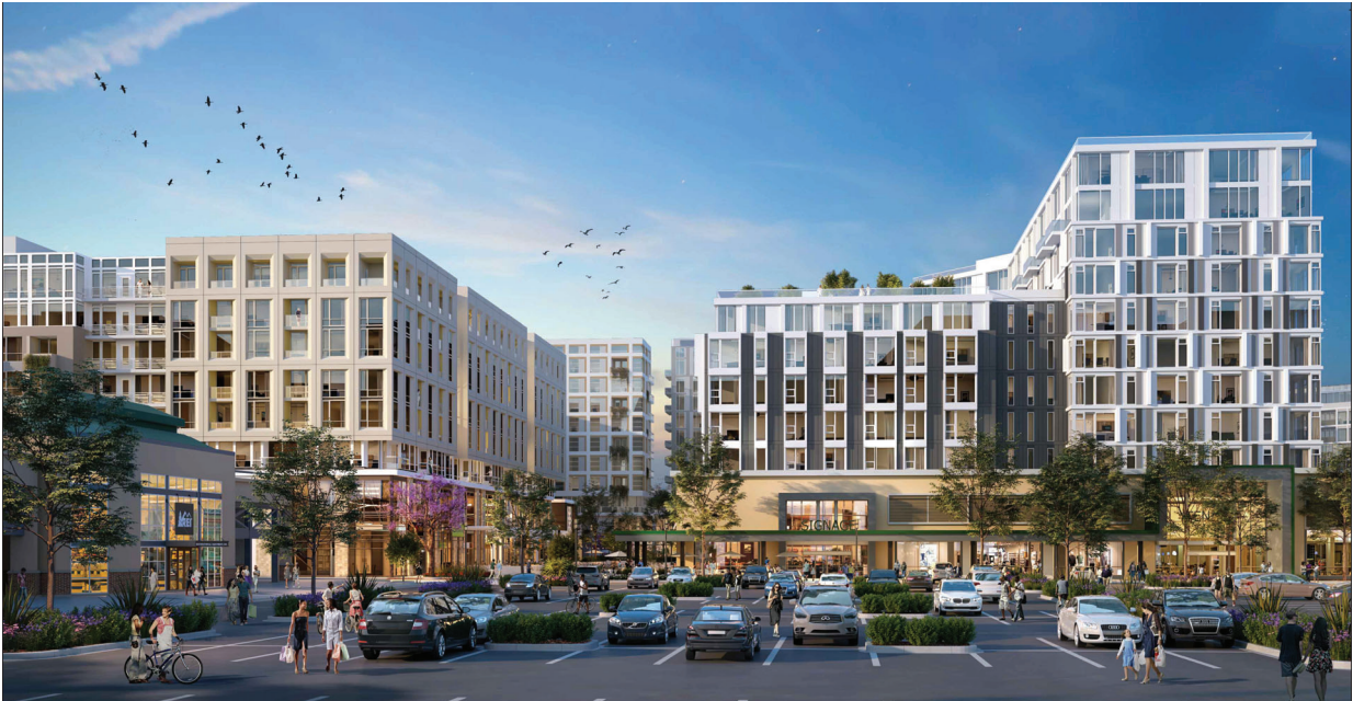
VIEW LOOKING WEST TOWARDS QUITO ROAD AND MAJOR COMMERCIAL TENANT
