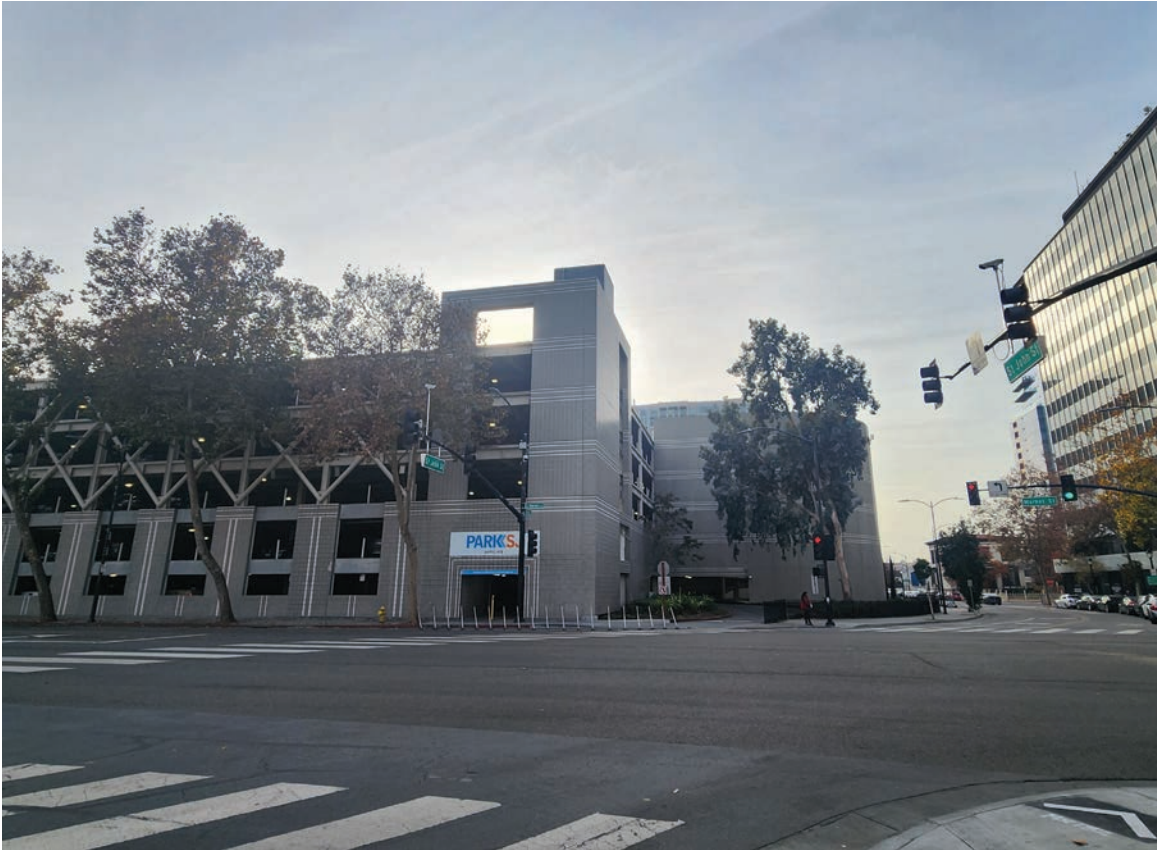
Photo 1: View of Market & San Pedro Garage from Market Street (looking west).
