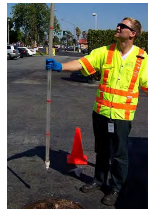
An inspector conducts a grease control device inspection.
