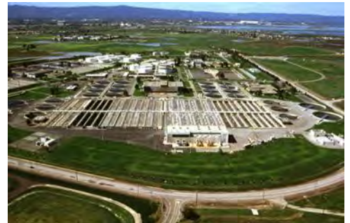
Aerial view of the Wastewater Facility
