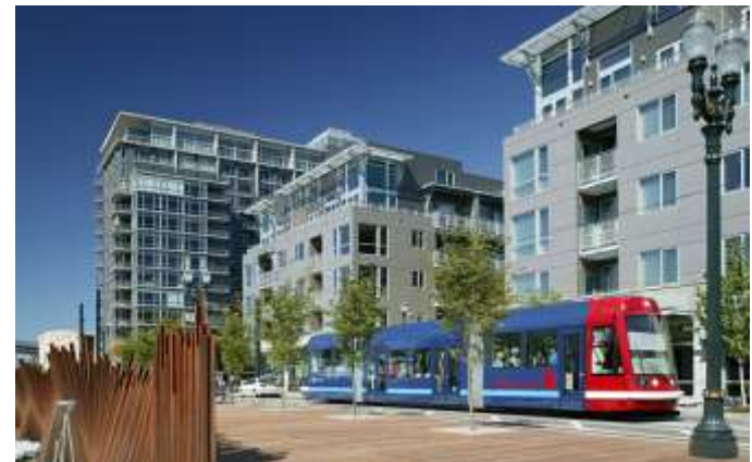
High-quality, compact, connected development
