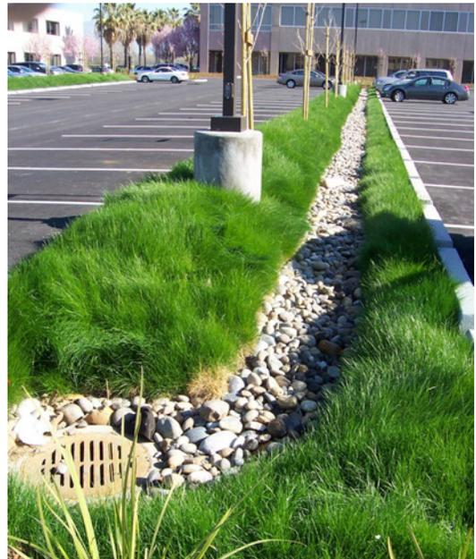
*Infiltration trench: a stormwater treatment control measure*
