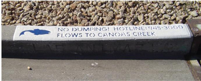
*Thermoplastic storm drain inlet marking on Chesbro Avenue*
