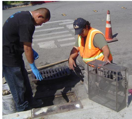
*Contractors installing a catch basin screen on Mt. Vista Drive for the structural trash pilot*
