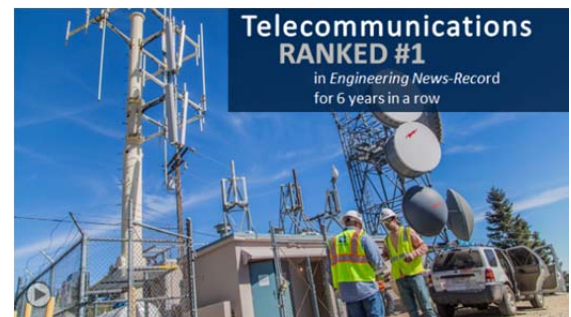
Figure 1 - Black & Veatch is a noted Telecommunication Systems planner and integrator, which means we design and assemble secure Smart City networks from the sensor to the cloud.
