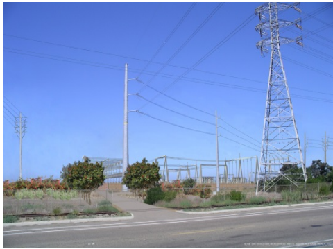
Substation rendering developed to support SDG&E's pursuit of CPUC approval of the project.
