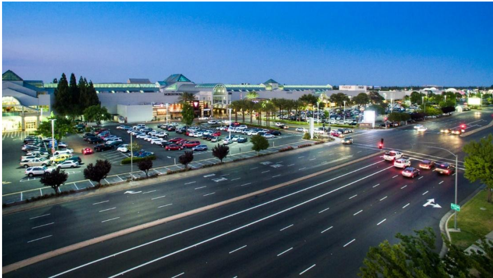
Arden Fair Mall after retrofit
