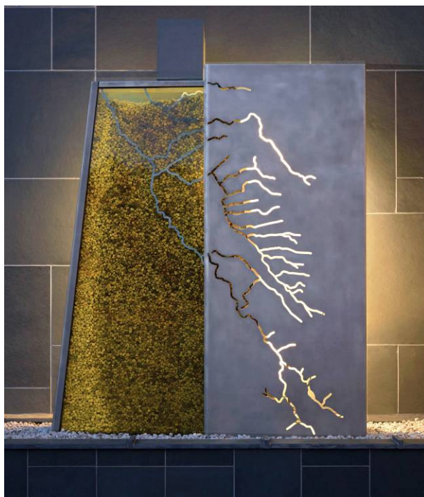
Vertical trickling filter: a stormwater treatment control measure and art exhibit at the Roosevelt Community Center
