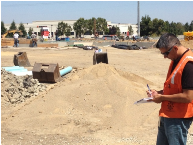
Environmental Inspector conducting an inspection for BMPs at a construction site
