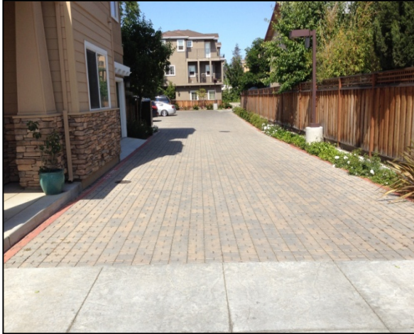
Permeable Pavement at a residential project site
