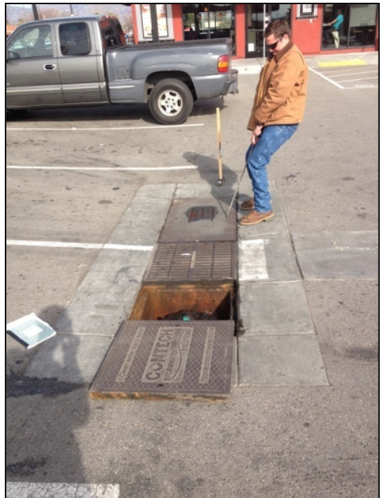
O&M Verification Program inspection of media inlet filter
