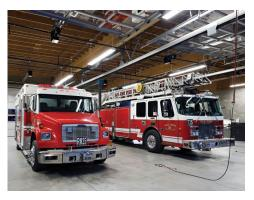
Energy was conserved by reducing the number of light fixtures in the fire station maintenance bays. Lights focused on the top of trucks was eliminated and remaining fixtures ensure the sides, front and rear of the trucks are well lit.
