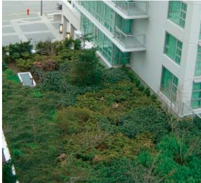
Green roofs improve insulation values, filter rainwater, and can be used as open space.
