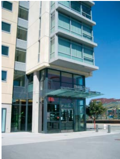
Building entrances should be clearly articulated and should face onto public streets or pathways.
