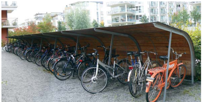
Well-designed, secure bicycle shelters can be integrated into common-use courtyards and can add to the design of a development.
