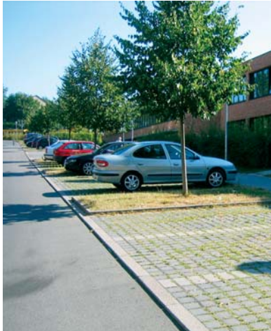
Permeable paving increases infiltration, reducing the amount of stormwater run-off.
