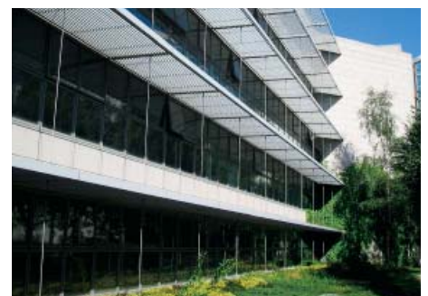
Utilize shading devices to minimize solar heat gain and optimize natural daylight use.
