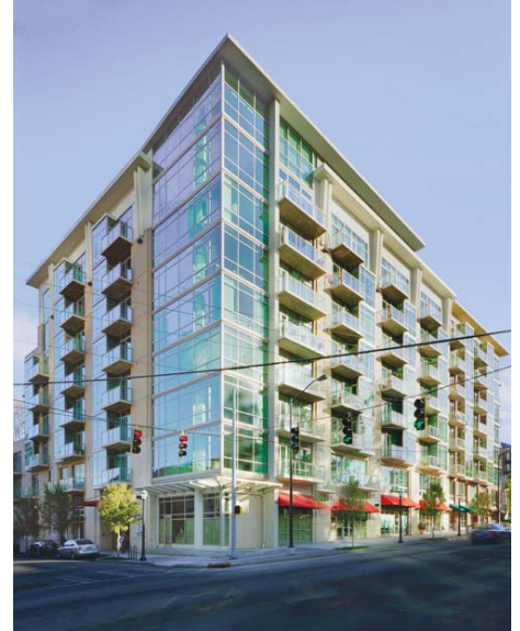
Use vertical façade modulation, floor height variation, and a mix of materials to create architectural interest.
