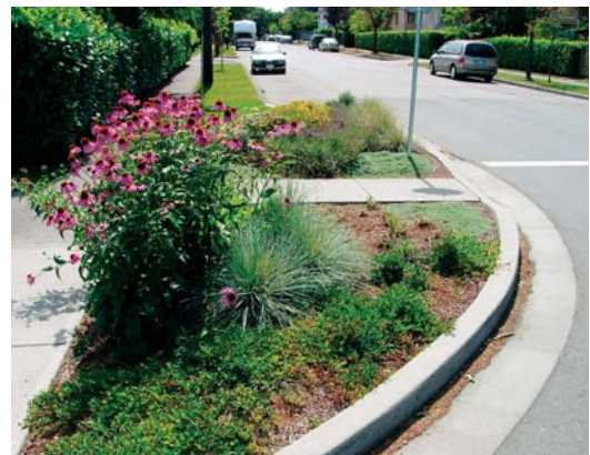
Bulb-outs, like this planted one, can help create a more pleasant pedestrian experience.
