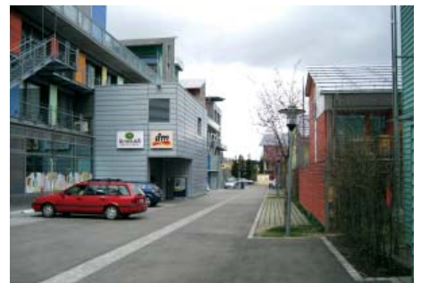
The back of a mixed-use building should be carefully designed. This example includes an alley, enclosed service areas, and a second store entrance.
