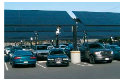
Solar panels utilized in parking lots can both generate electricity and provide shading for cars.
