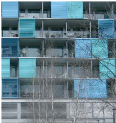
Exterior shading elements can be used as a key design feature of a building façade.
