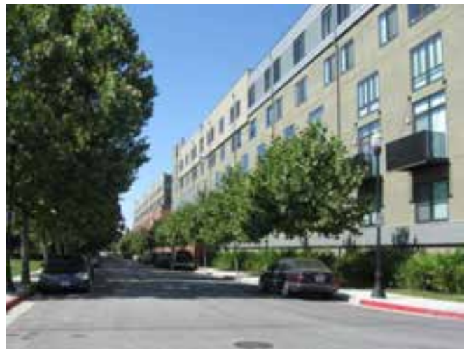
22) Plant 51, north of Cahill Park
