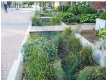
Bioswales retain rain water and reduce the impact on the storm water system. If designed well, they can improve and green the streetscape.
