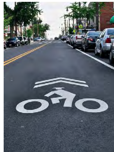
A Class III bike way is marked with a sharrow to indicate that the street is shared by cyclists and motorized traffic
