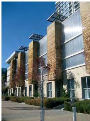
Above-ground parking garages fronting on a street or public pathway should have ground-floor uses such as retail or office space.
