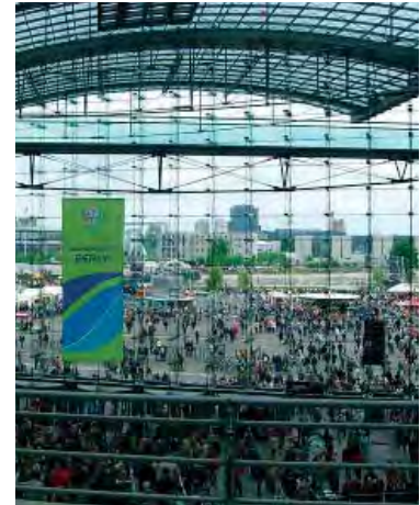
The station and the station area will be the place where the city welcomes visitor, employees and residents alike.
