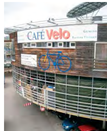
Stand-alone bike parking and repair facilities can include other uses such as car share or a café.
