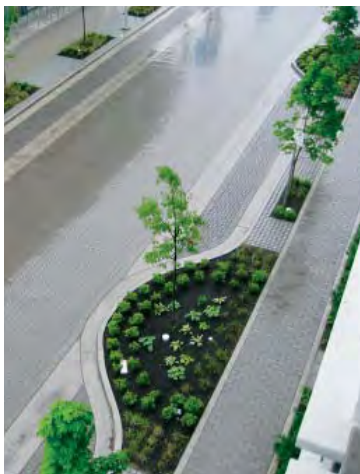
Provide generous bulb-outs for street trees and pay attention to detailing for curbs, drainage, and pavement.
