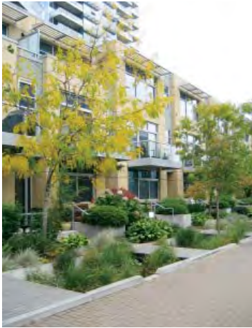
Residential buildings should have a fine-grained articulation through porches, balconies and transition zones, particularly when fronting on a street or public pathway.
