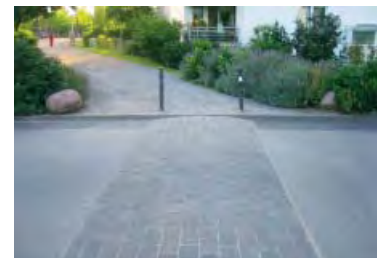
Speed tables work to both slow down traffic as well as provide a clear pathway way for pedestrian travel. They can be adopted for both residential and urban conditions.
