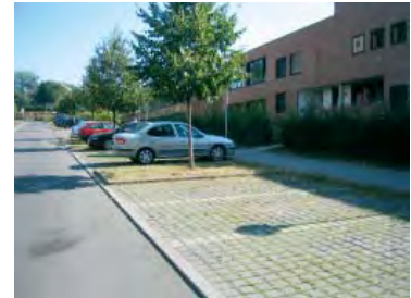
The use of pervious materials in surface parking areas increase water infiltration and decrease the heat island effect. Different pavement for street parking also visually narrows the street.
