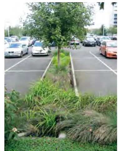
Provide planting strips in and around the perimeter of surface lots to increase water infiltration and add visual interest.
