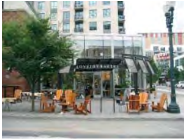
Prominent design of ground floor retail contributes to high visibility and increases activity on the street.
