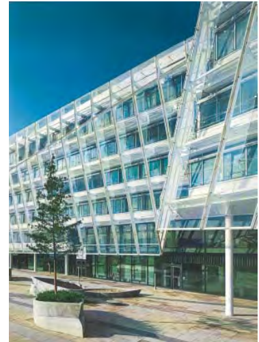
Double skin façades can provide natural ventilation and improve insulation in office buildings.
