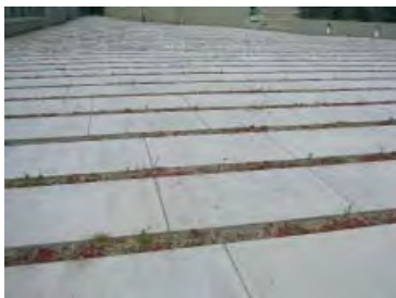
Permeable paving can help to reduce urban runoff while creating a distinctive look.
