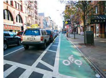
Separated and colored Class II bike lanes improve visibility and safety for cyclists (example: New York City)
