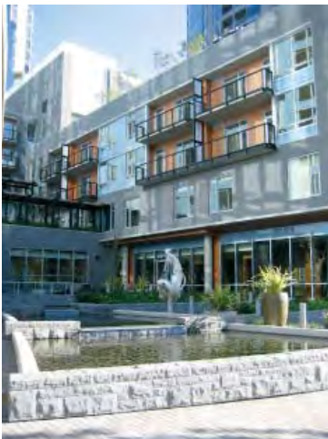
Buildings can be oriented perpendicular to the street to frame open spaces.
