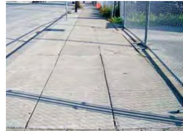
Existing Conditions, Montgomery Street Source: Fehr & Peers, 2010
